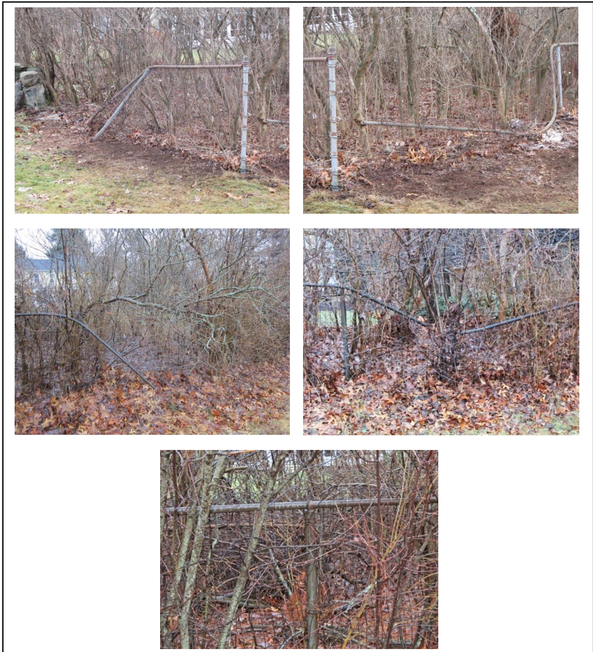
Figure 3-23. Examples of damage to the woven wire fence along the southwest side of the Old Section. Upper two rows of photos show damage to the woven wire and fence structure caused by fallen trees. These sections will require replacement. Note also the dense scrub vegetation that must be removed from around the fence. The lower photo shows a detail of intact fencing.
