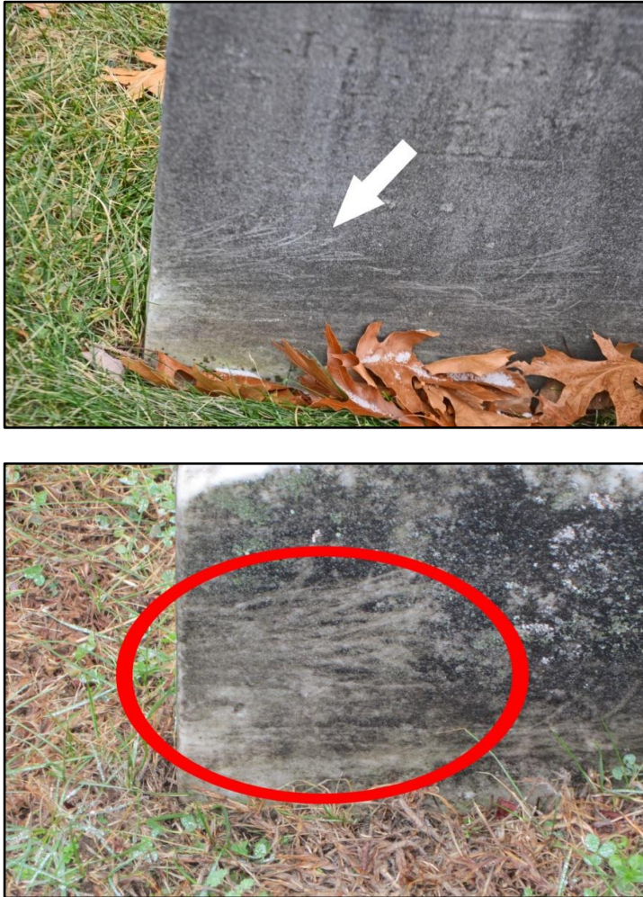
Figure 3-35. Nylon trimmer damage caused by improper operation and the use of string that is too heavy for the delicate stones.
