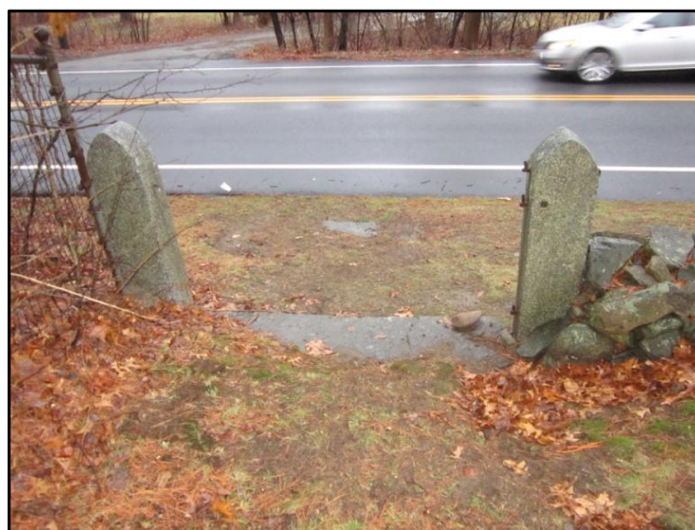
Figure 3-15. Pedestrian gates. The upper photo shows the central gate with pintles in the southern post. The lower photo shows the southern gate with pintles in both columns, indicating a double gate.
