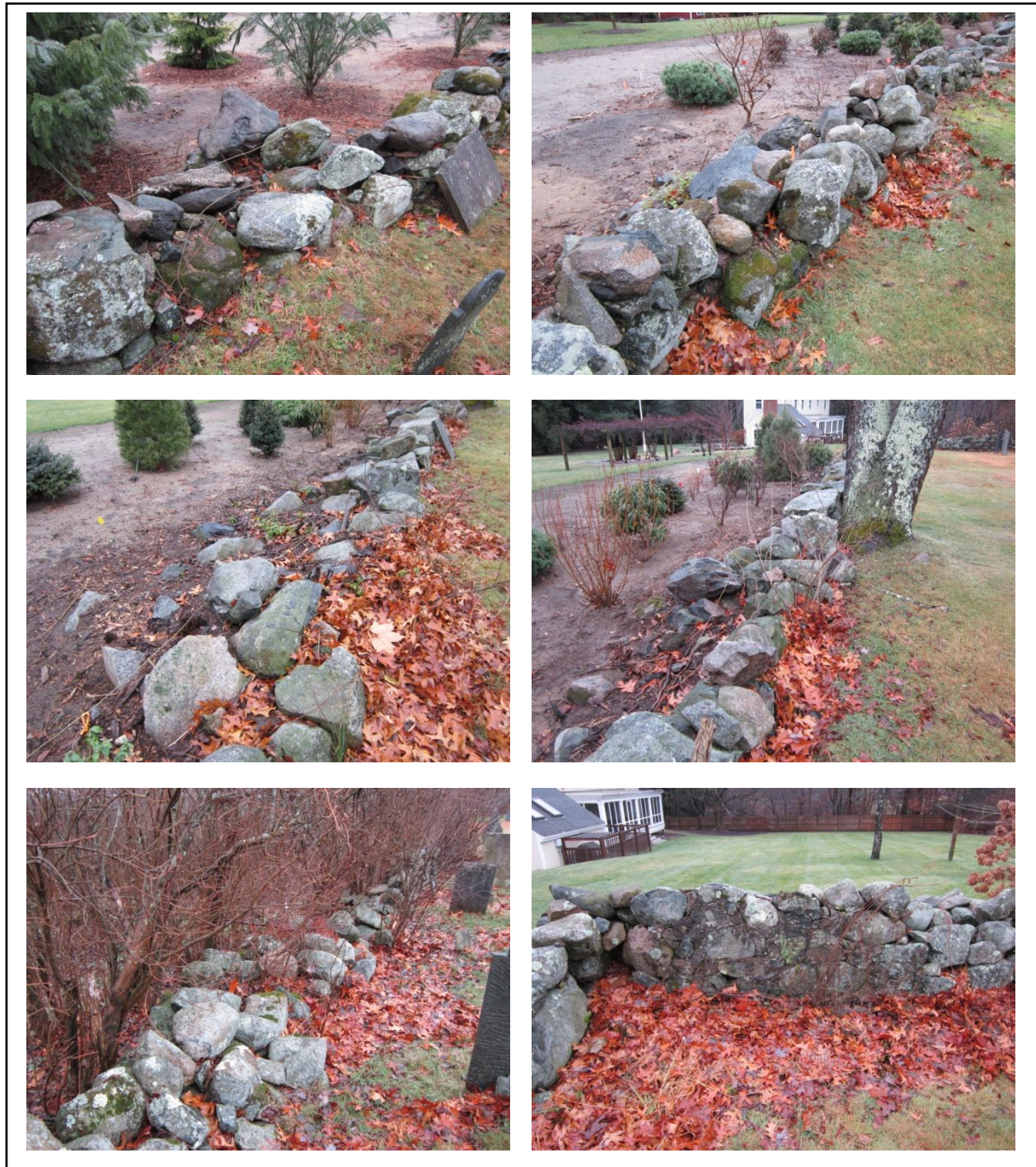
Figure 3-22. Examples of damage to the stone wall on the east side of the Old Section. The upper row shows examples of failing wall, with toppled stones. The middle left photo shows the wall barely protruding from the grade with fallen stones partially buried. The middle right photo shows a tree intruding into the wall. The lower left photo shows scrub vegetation intruding into the wall as well as collapsing stones. The lower right photo shows a wall section poorly pointed with a hard Portland cement mortar.
