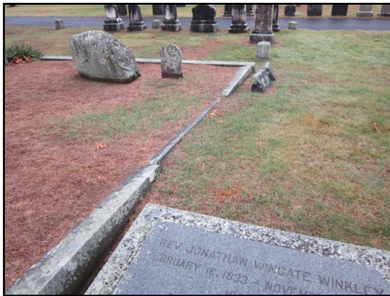
Figure 3-45. Displaced and sinking curbs are common, especially in the Stoney Section.
