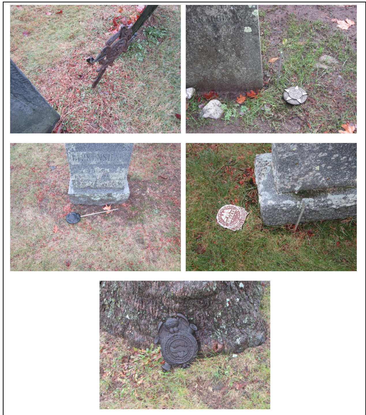
Figure 3-44. Damaged and orphaned emblems in North Cemetery. Upper left is an example of a broken shaft in the Old Section. Upper right shows a damaged emblem from the Lovell South Section. Middle left shows a fallen emblem in the Lovell Section. Middle right shows a damaged emblem from the Lovell Section. Bottom image shows an orphan emblem from Section A. Failure to repair or replace these military emblems is not only disrespectful, but will result in many being stolen.
