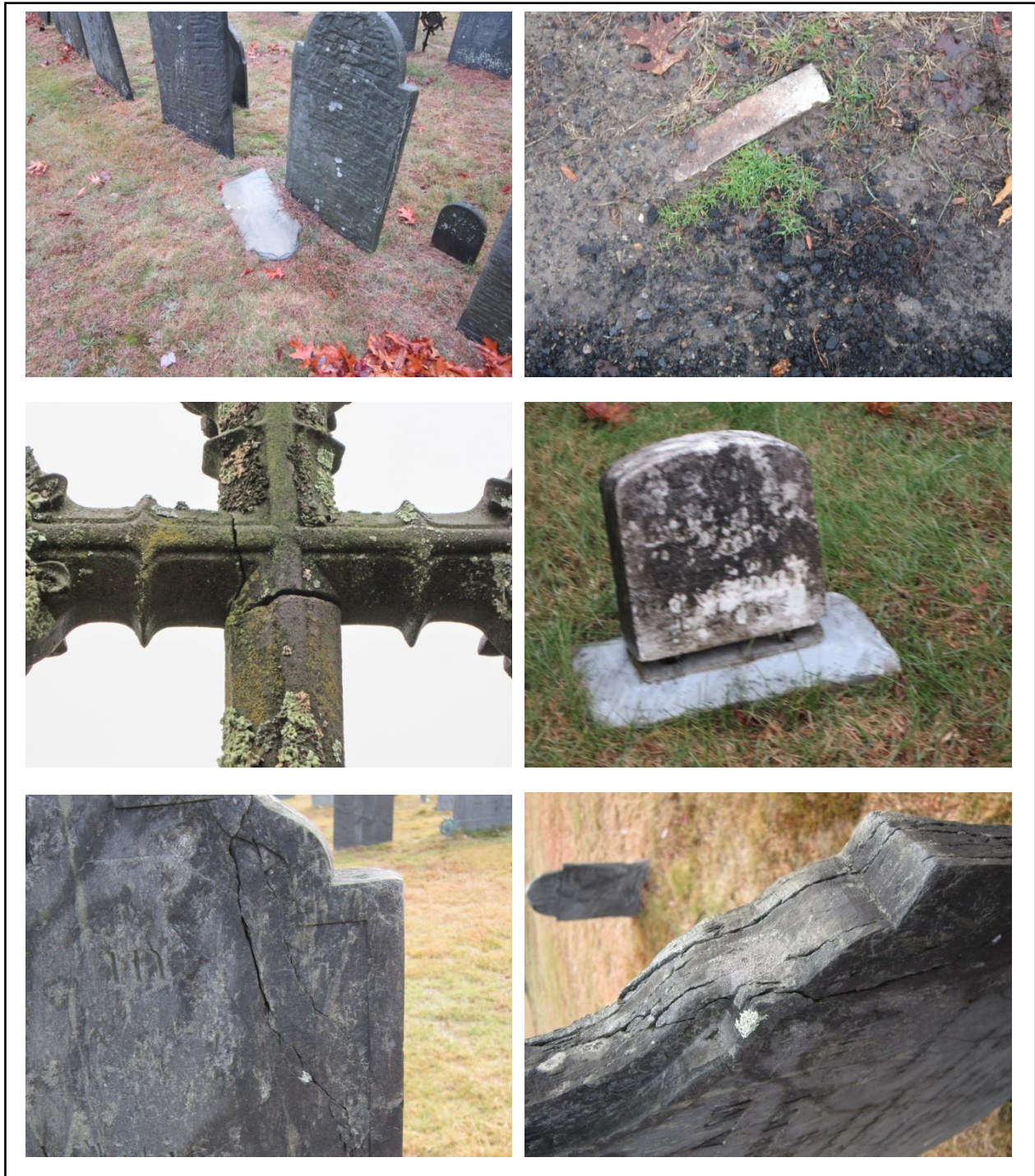
Figure 3-52. Examples of damaged stones. Upper left shows a stone out the ground (Stoney Section). Upper right shows a broken stone (Stoney Section). Middle left shows a broken sandstone cross with heavy lichen (Stoney Section). Middle right shows unattached die on base (Stoney Section). Lower left shows a cracked slate (Old Section). Lower right shows severe spalling of a slate stone (Old Section).
