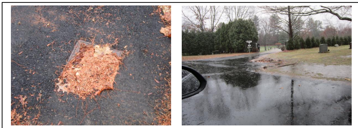
Figure 3-48. Issues with drains in the Cemetery. The photo on the left shows a drain clogged by leaves and other debris. On the right is a photo of a largely ineffectual drain with soil piled up around it, causing localized flooding or ponding of water in the cemetery.
