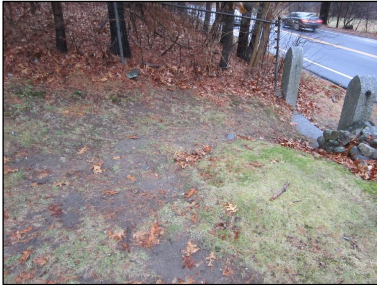
Figure 3-16. Erosion at the southern pedestrian gate fronting Old Sudbury Road.
