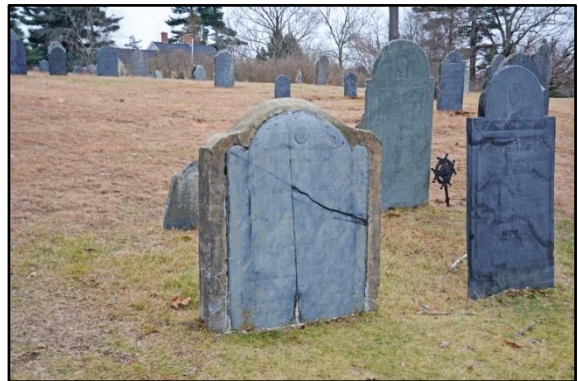
Figure 3-49. Poor repairs. In the top photo a silicon caulk has been used in an effort to adhere a broken slate stone. In the lower photo a slate stone has been encased in a hard Portland cement.
