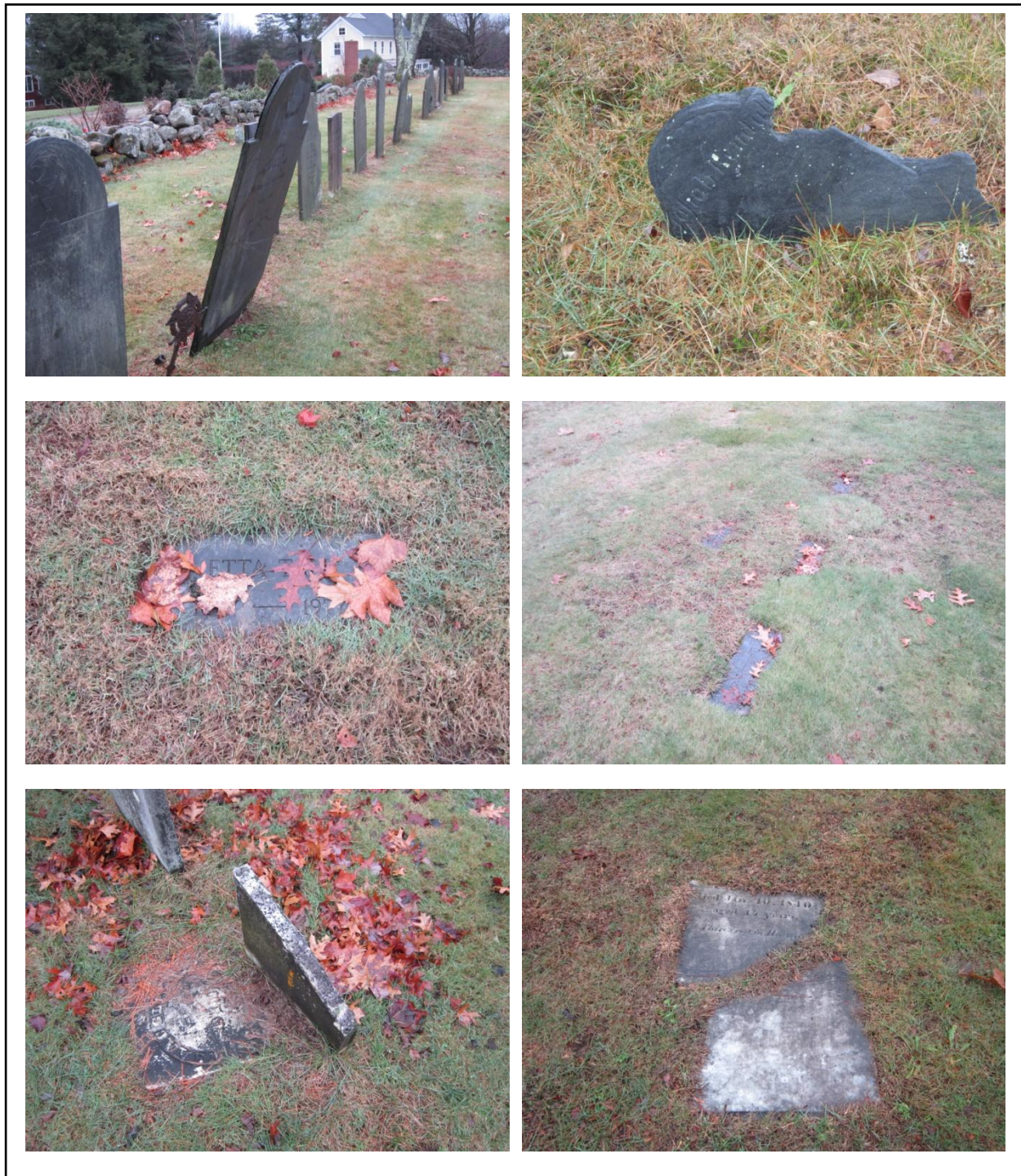
Figure 3-51. Examples of damaged stones. Upper row shows severely tilted stones, both the Old Section. Middle row shows sunken markers in the Jewish Section (left) and Lovell Section (right). Lower row shows broken stones in the Old Section (left) and Lovell Section (right).
