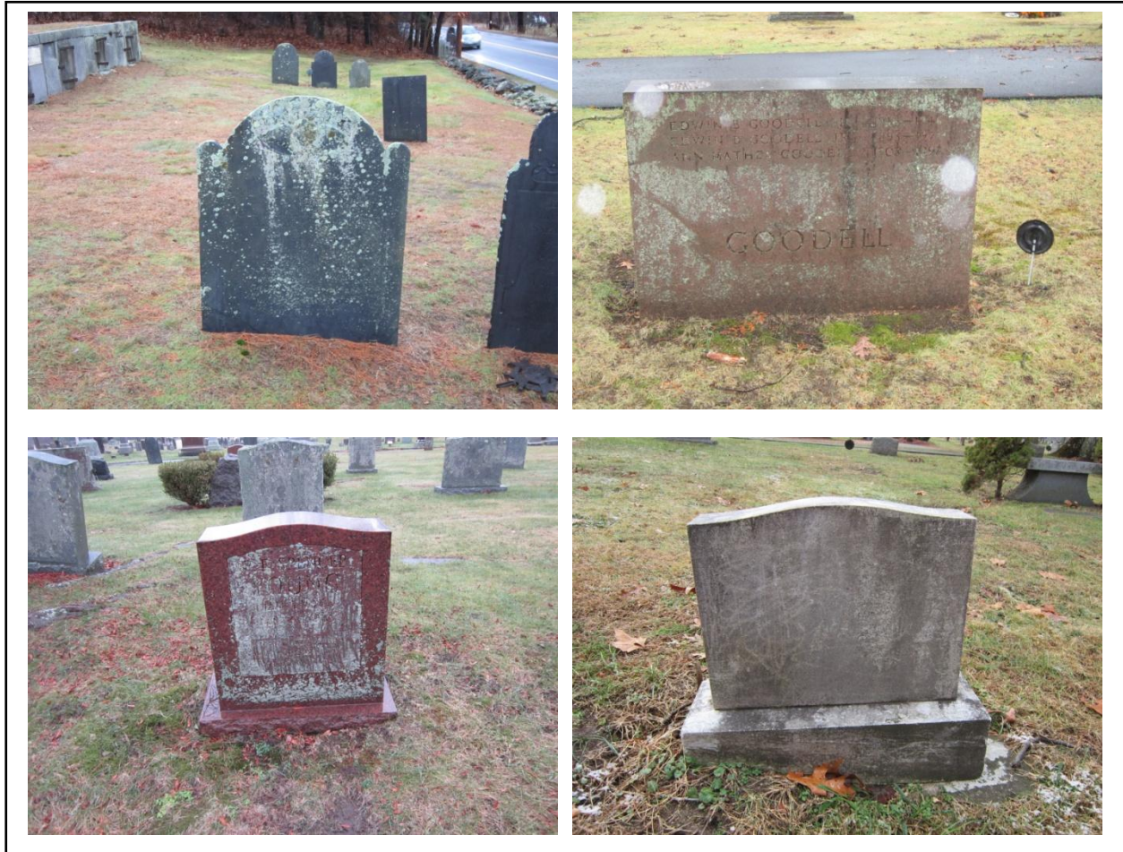
Figure 3-53. Cleaning Issues. Upper left photo shows typical extensive development of lichen on many stones at North Cemetery. Upper right and lower left both illustrate improper efforts to clean just names, probably for genealogical research. Lower right photo shows a marble stone incorrectly cleaned with a pressure washer (notice the streaks, especially on the left side of the die).
