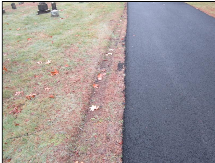
Figure 3-11. Damage to roadside by car leaving the road to park.
