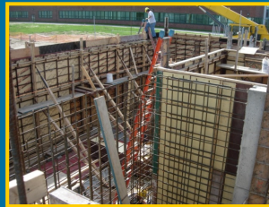
Steel Prior to Inspection
