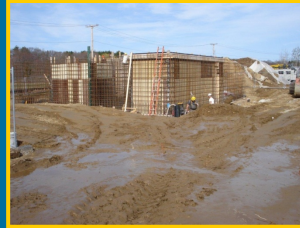
Steel & Form Work
