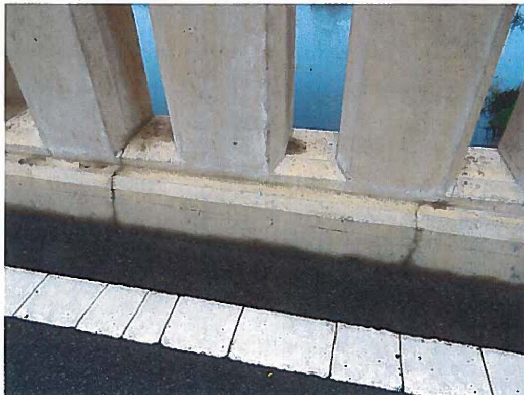
Photo 2: East bridge rail base near South end.
