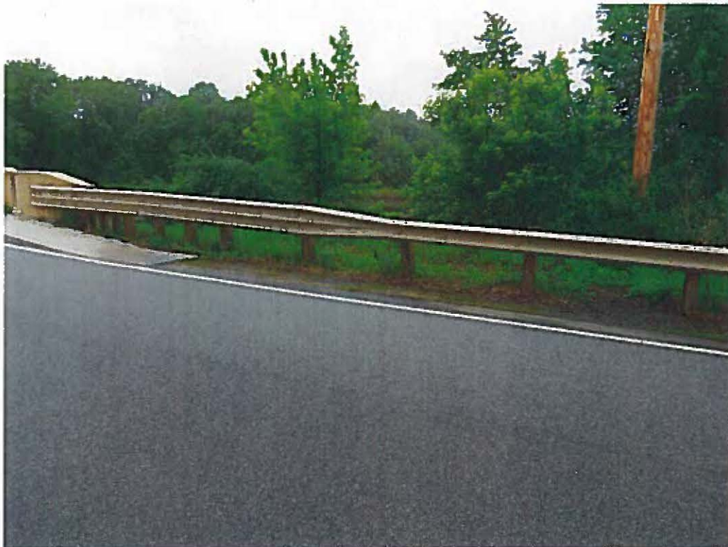
Photo 4: Northwest approach guardrail.
