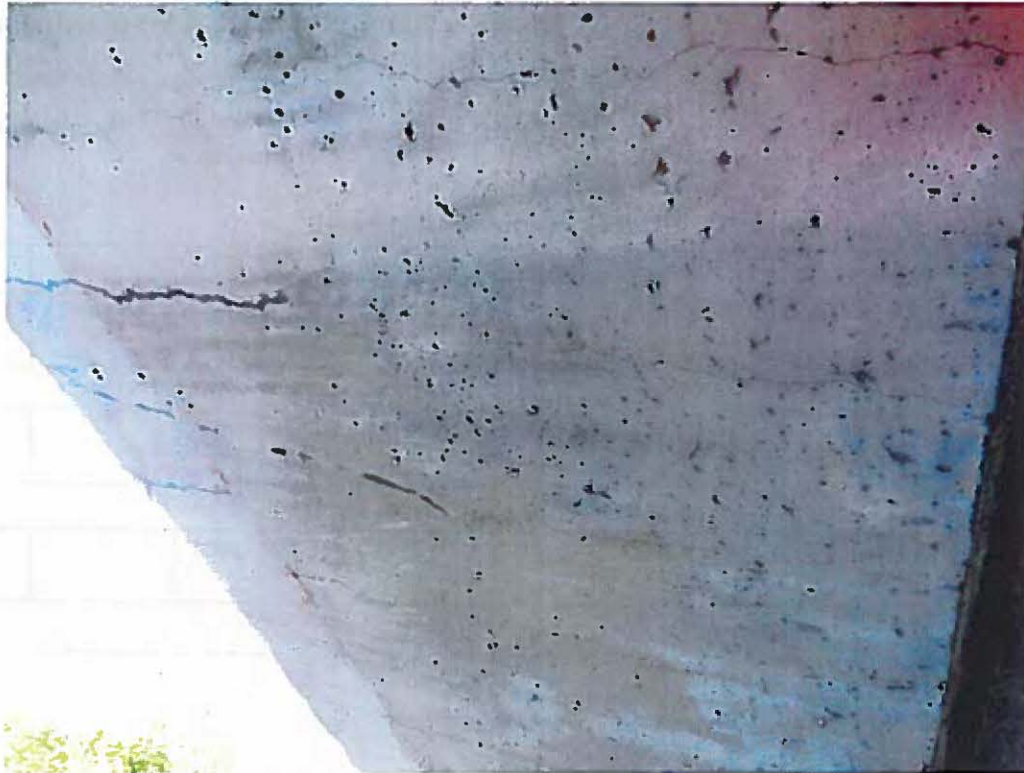
Photo 3: Arch segment #1 near midspan.
