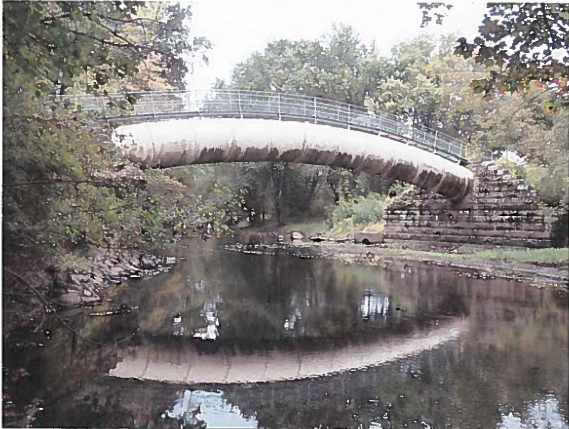
Weston Aqueduct Sudbury River crossing
