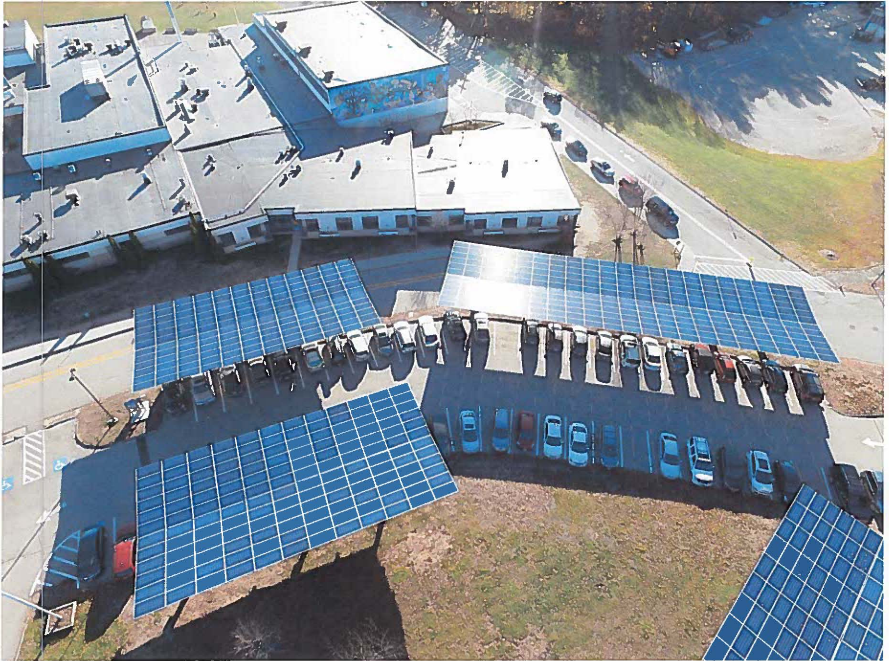
Wayland Middle School, System Type: Carport, Solar Panel Quantity: 756, DC Capacity: 238 kW, AC Capacity: 208 kW
