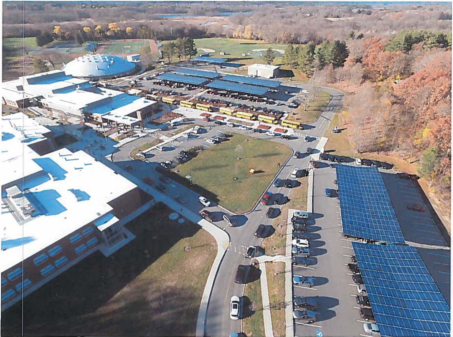
Wayland High School, Carport, Solar Panel Quantity: 1,938, DC Capacity: 610 kW, AC Capacity: 500 kW
