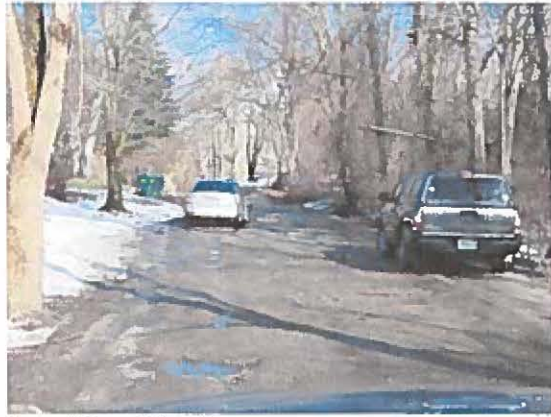
Potholes on unpaved portion of Heard Road
