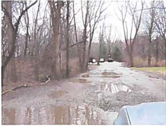
Potholes on unpaved portion of Heard Road
