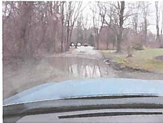
Ponding at end of paved portion of Heard Road
