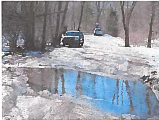
Ponding at end of paved portion of Heard Road
