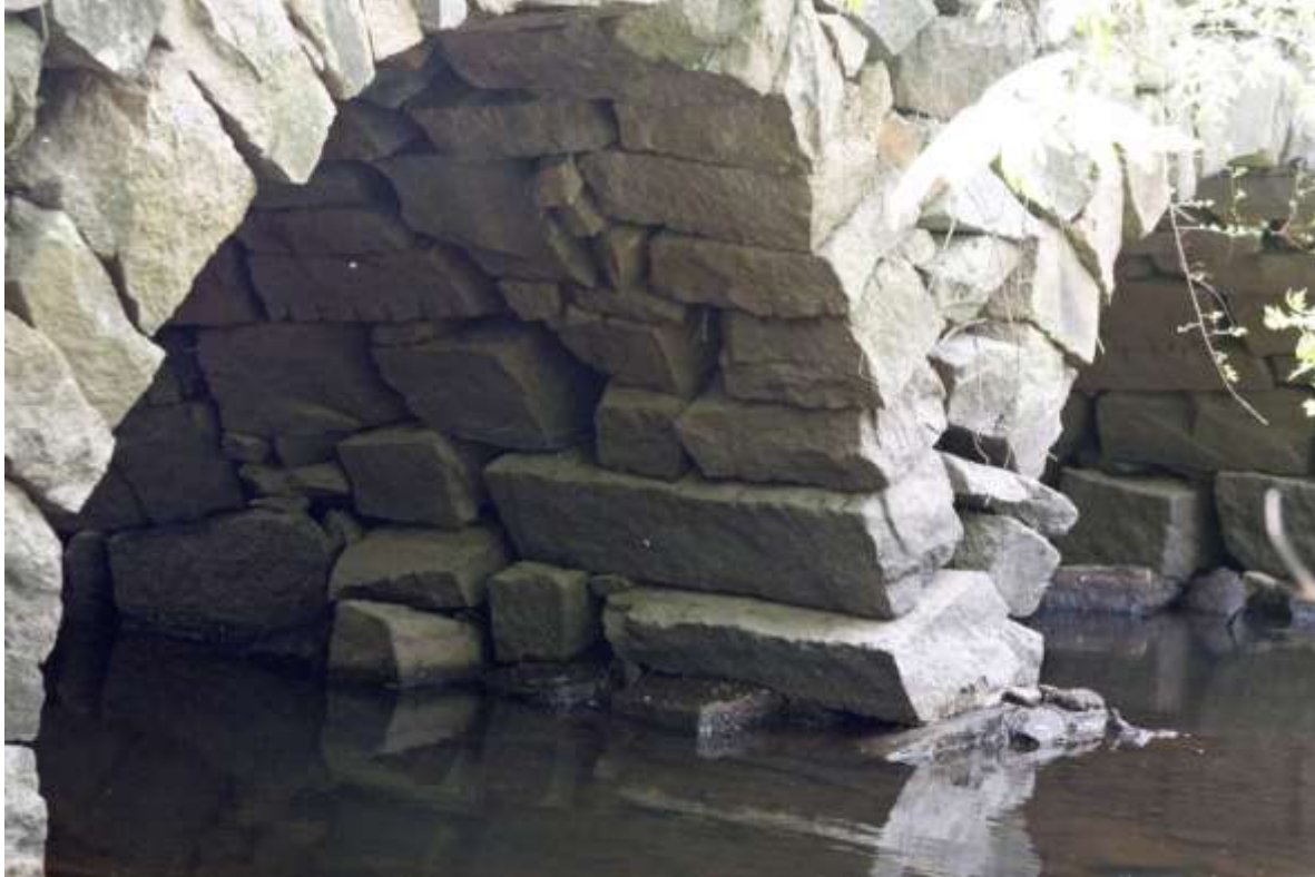
Stone's Bridge – underside of two arches
