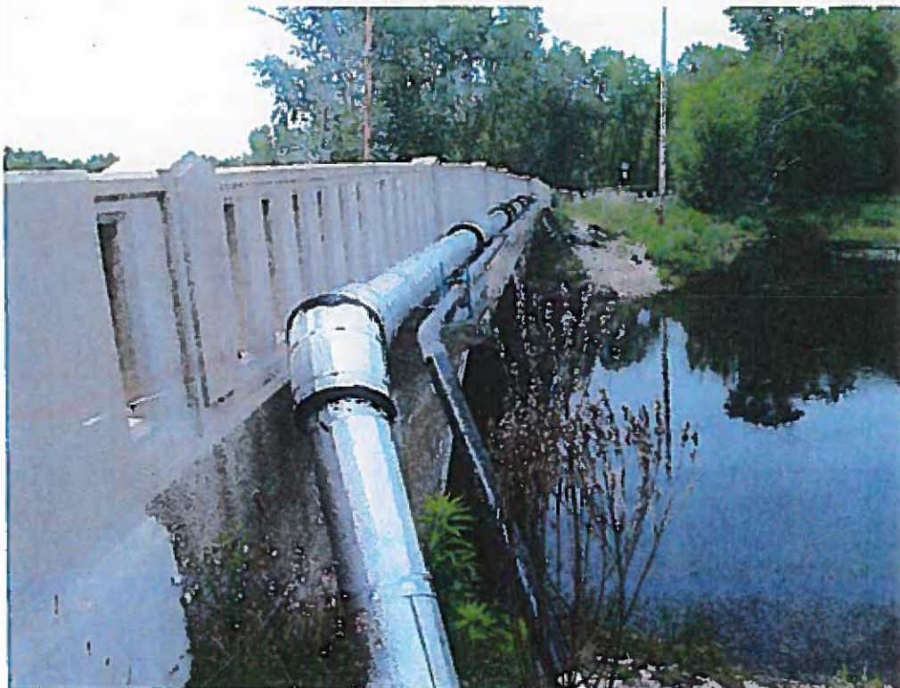
Photo 2: Utilities attached to South spandrel wall.
