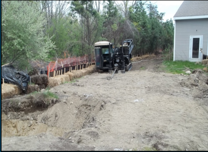
Force Main Outfall Installation – Horizontal Directional Drilling Rig Set Up
