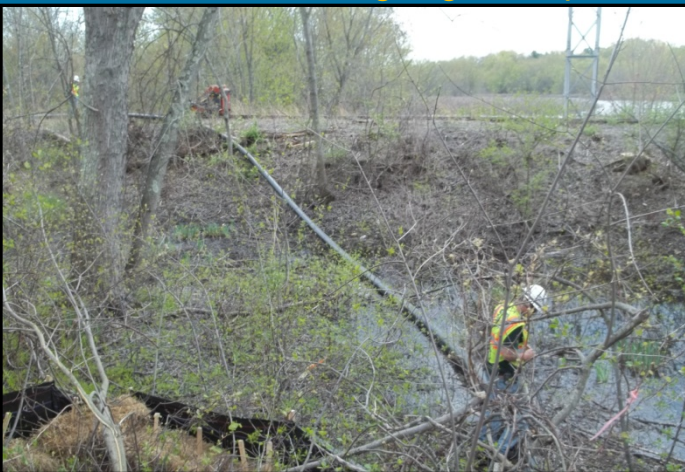
Fused HDPE Force Main Pipe
