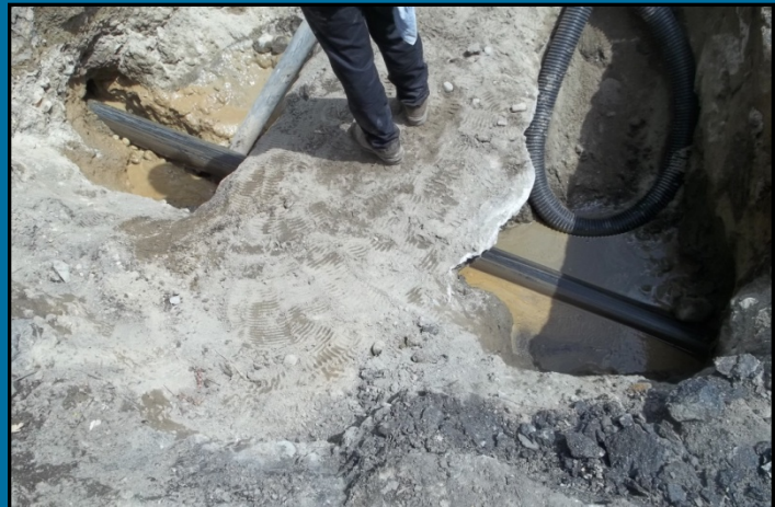
HPDE Force Main Pulled Underneath Fiber Duct Bank off of Route 20
