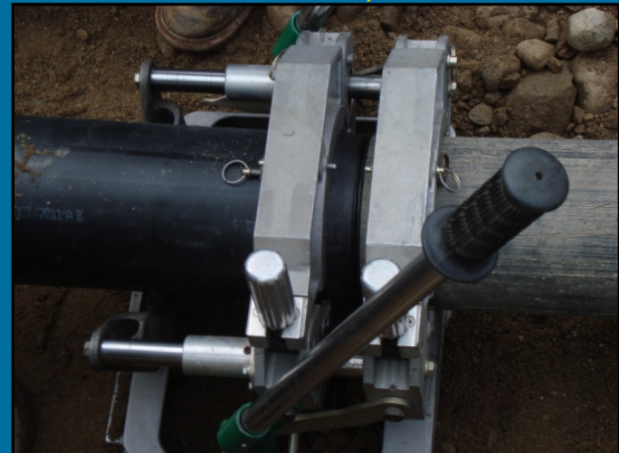
Heat Fusion Joining of HDPE Force Main Piping
