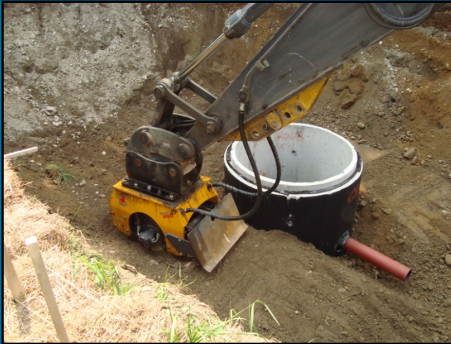
Force Main Outfall Pipe and Structure Installation – Open Cut Methods
