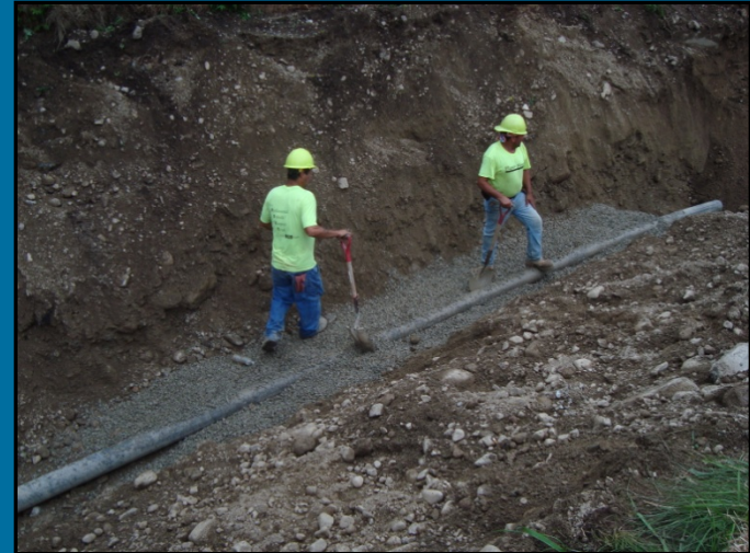
Force Main Outfall Pipe Installation
