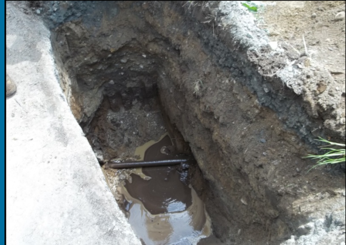
Horizontal Directional Drilling Bore at Exit
