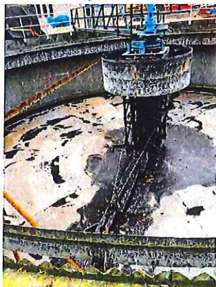
Secondary Clarifier No. 2 Ready for Equipment Demo.
