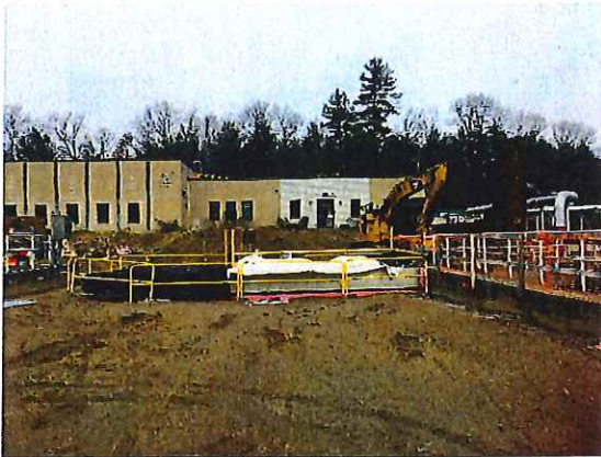
Secondary Clarifier No. 2 Ready for Equipment Demo.
