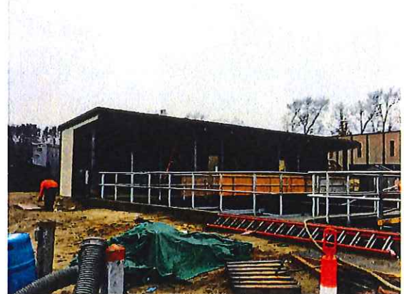
New Primary Clarifier Canopy 02/2019
