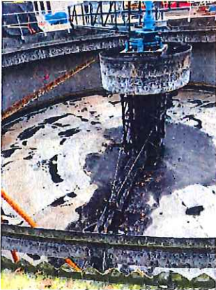
Secondary Clarifier No. 2 Ready for Equipment Demo.
