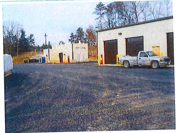
New Septage Receiving & Garage Paved 12/2018
