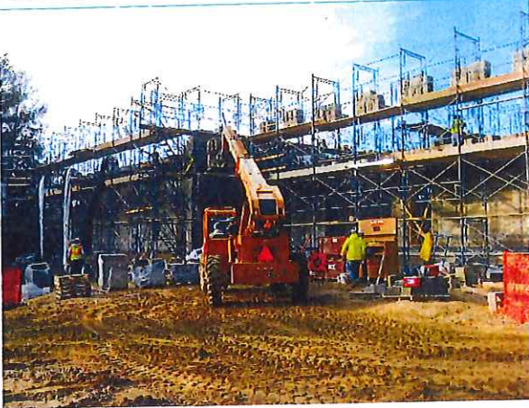
New Aeration Splitter Box Wall Forms 11/2018
