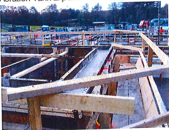
Aeration Tank Expansions Catwalk Poured 11/2018
