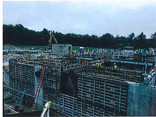
New Filter Building Walls 9/2018
