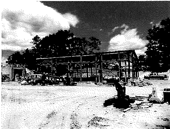
New Septage Receiving & Garage
