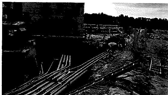
Secondary Electrical Banks
