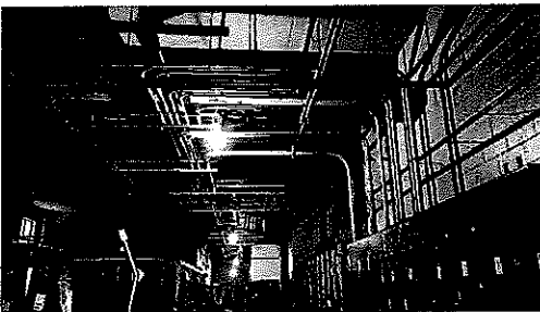
New MCC and Conduit in Process Building
