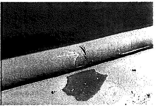
Defect #3 – Splits in expansion joint Defect #3 – Splits in expansion joint
