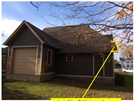
Install Ice & Water on lower roof sections (both sides) on the backside of the Carriage House. Install Ice & Water on both sections, plus six feet up on next section. See Specifications
