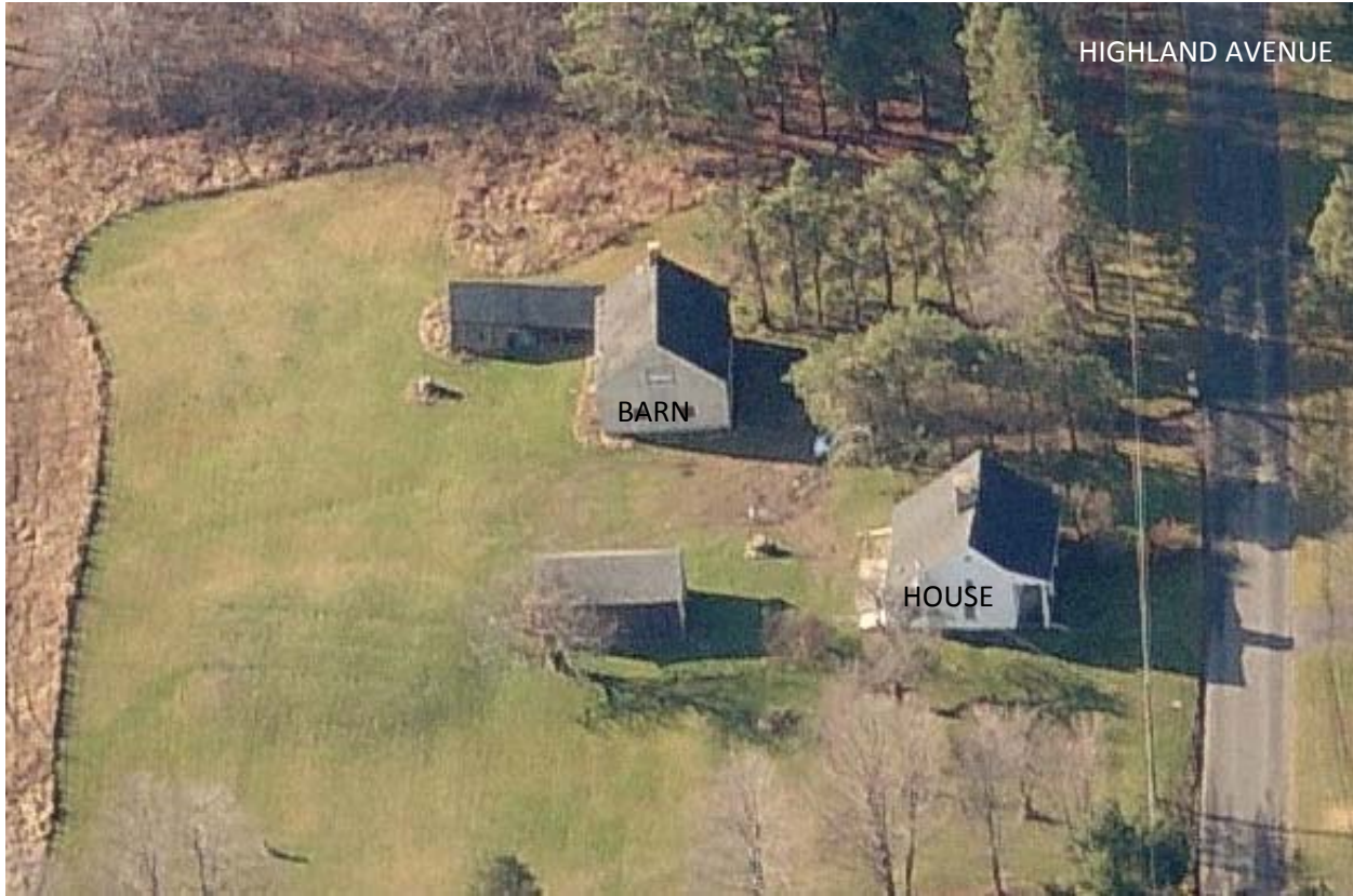
AERIAL VIEW LOOKING WEST (CLOSE UP) – Area of Site Survey
