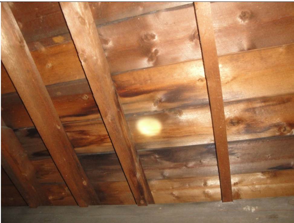
Photo R4 08/13/15 Photo Location: Attic interior.
