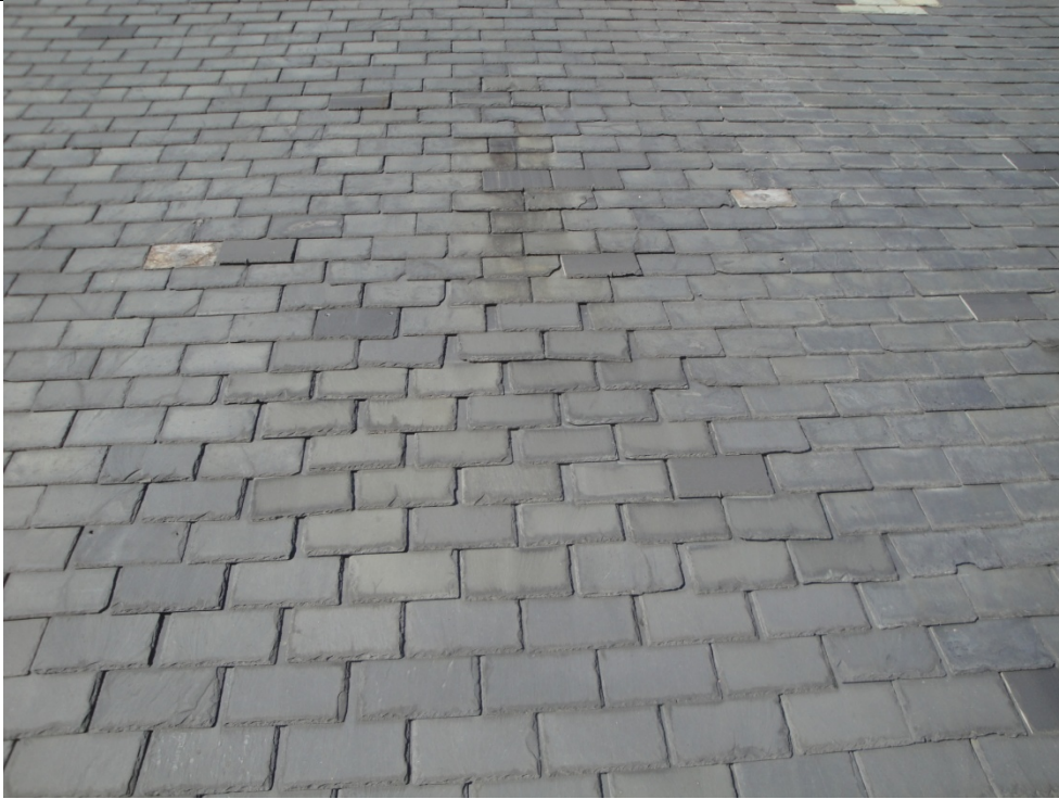
Photo R15 08/33/15 Photo Location: Upper main hip roof.
