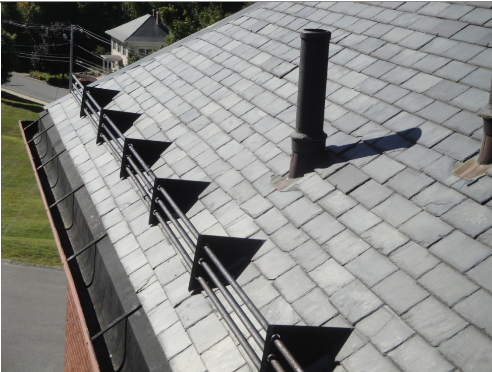
Photo R10 08/13/15 Photo Location: Northeast elevation.
