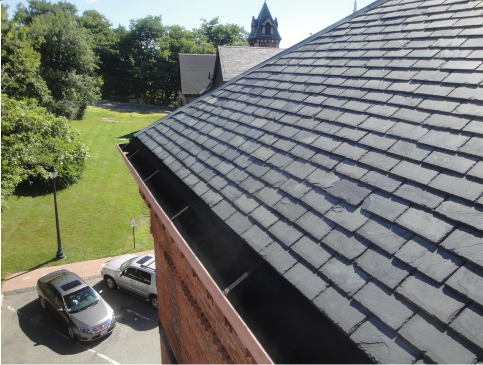
Photo R9 08/13/15 Photo Location: Upper main roof northwest elevation.
