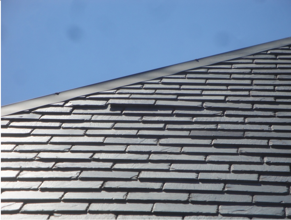
Photo R17 08/13/15 Photo Location: Upper main hip roof.
