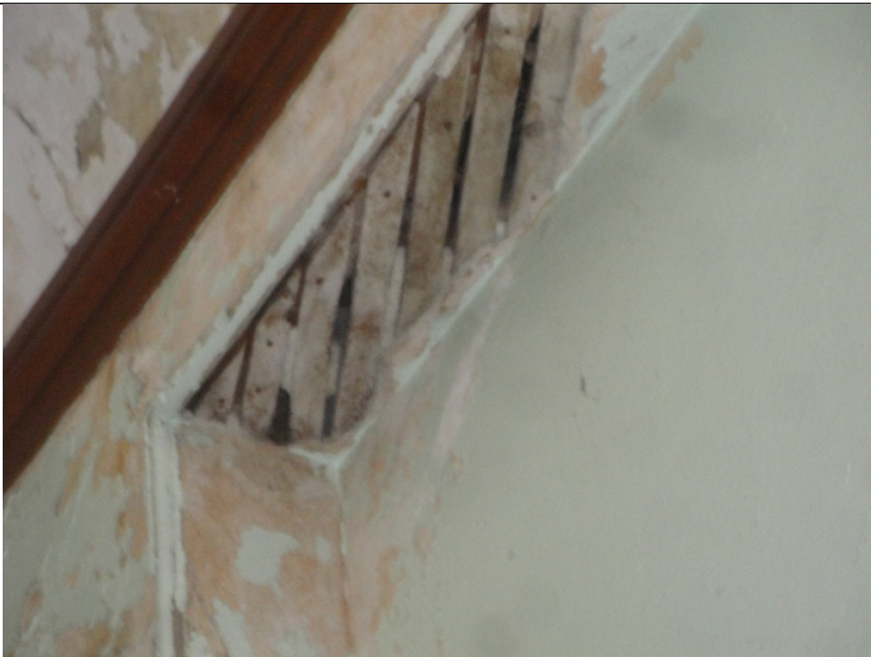
Photo R6 08/13/15 Photo Location: Interior upper floor.
