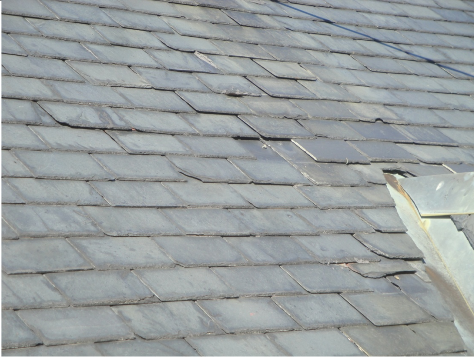
Photo R21 08/13/15 Photo Location: Upper main hip roof.
