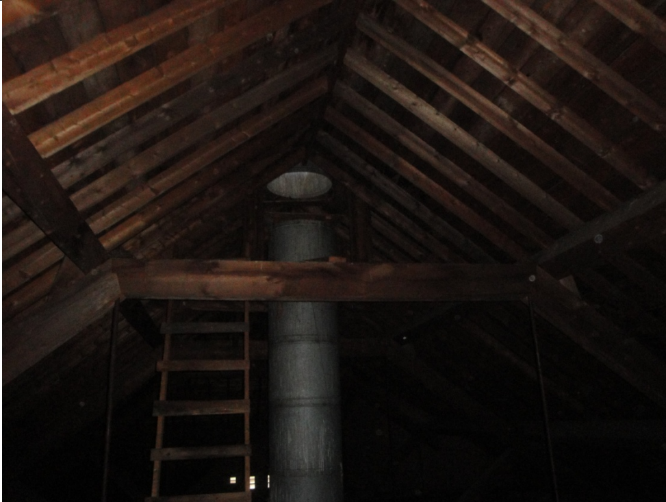
Photo R3 08/13/15 Photo Location: Attic interior.
