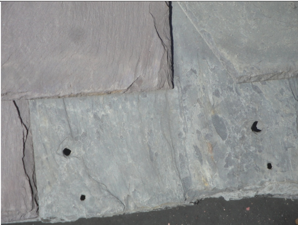
Photo R18 08/13/15 Photo Location: Upper main hip roof.
