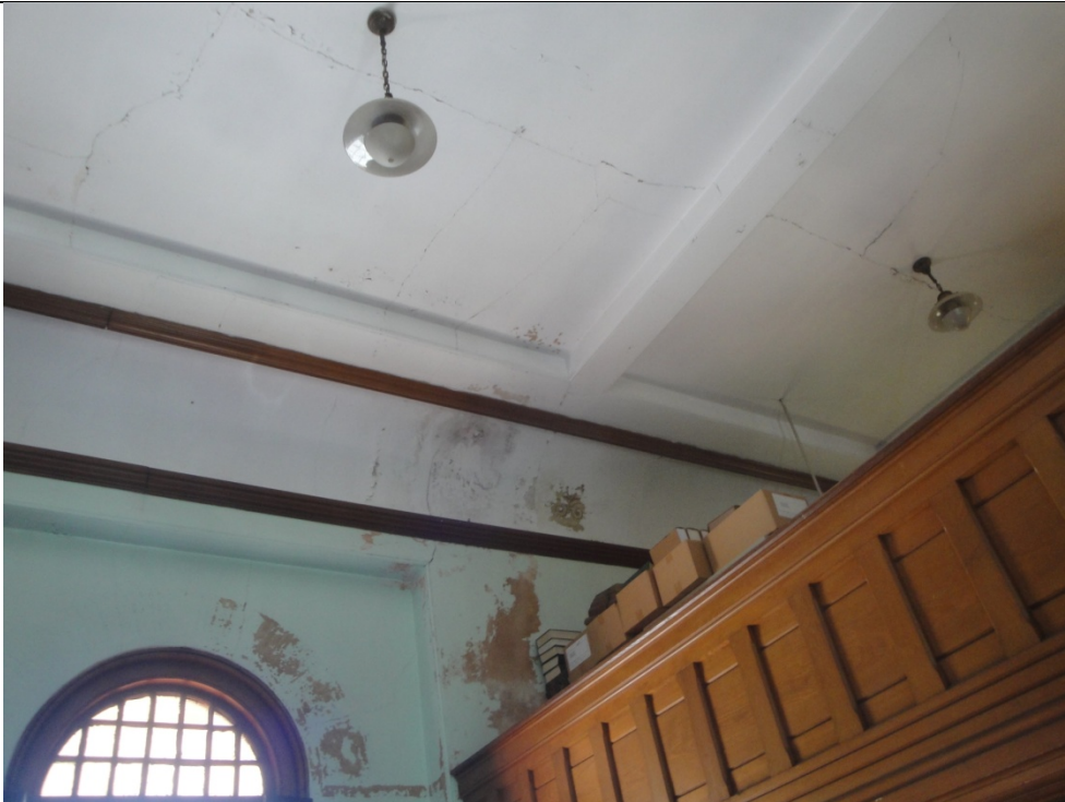
Photo R5 08/13/15 Photo Location: Upper floor.
