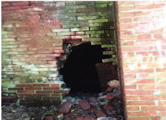
Masonry damage on Northwest wall
