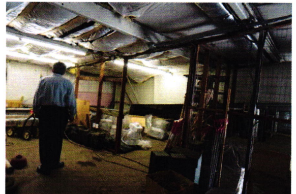
DPW Mezzanine Loft – note vapor barrier failures
