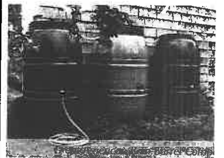
An example of 60-gallon rain barrels. Some communities in MA offer a rain barrel program that offers significant discounts to residents.
