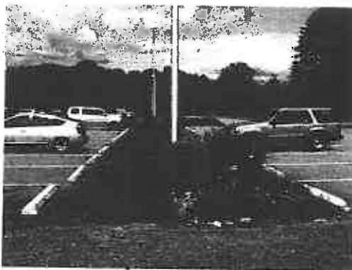
Bioretention strips filter parking lot runoff.
