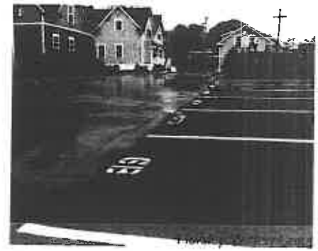
This parking lot in Narragansett, RI shows traditional asphalt on the left, where puddles have formed, and permeable pavement on the right, where it has soaked through.
