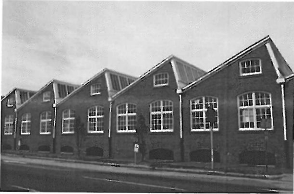
Figure 65: Building forms that reflect an industrial heritage
