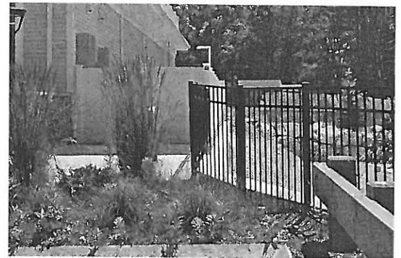
Figure 23: Integrated and screened utilities
