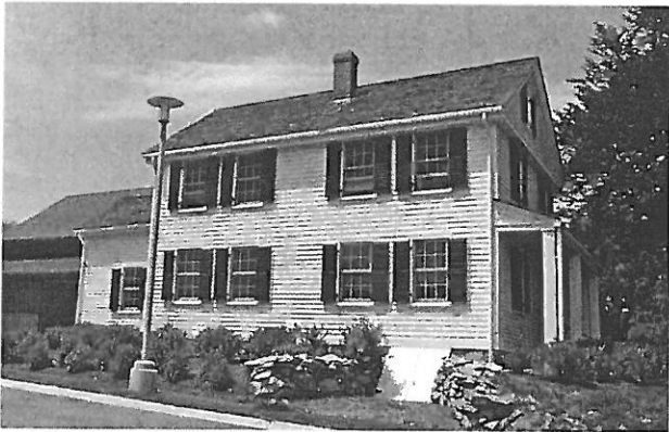
Figure 35: Traditional New England roof typologies are encouraged to reinforce a regional sense of place
