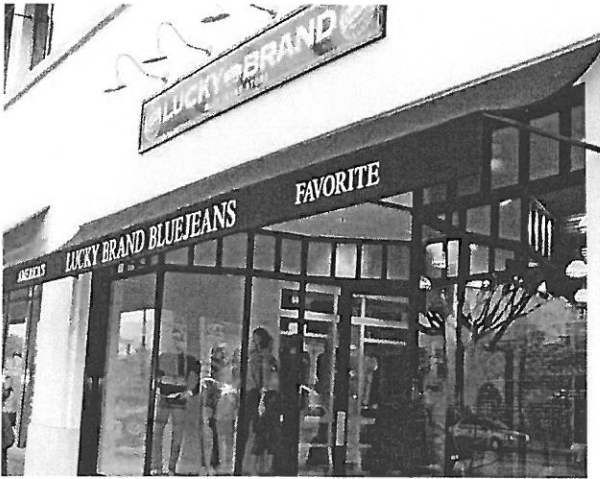
Figure 46: Awning is opaque and integrated into the building façade
