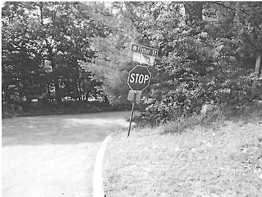
Leaning sign and no pavement markings
