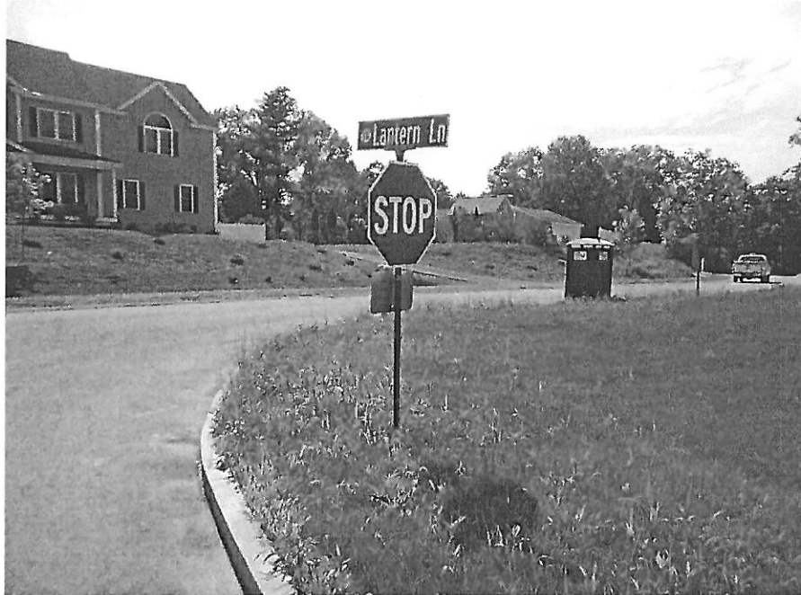
Incorrect sign height and no pavement markings
