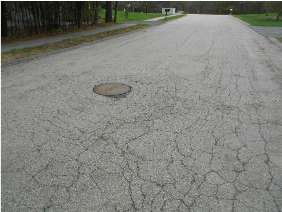
Roadway Cracking
