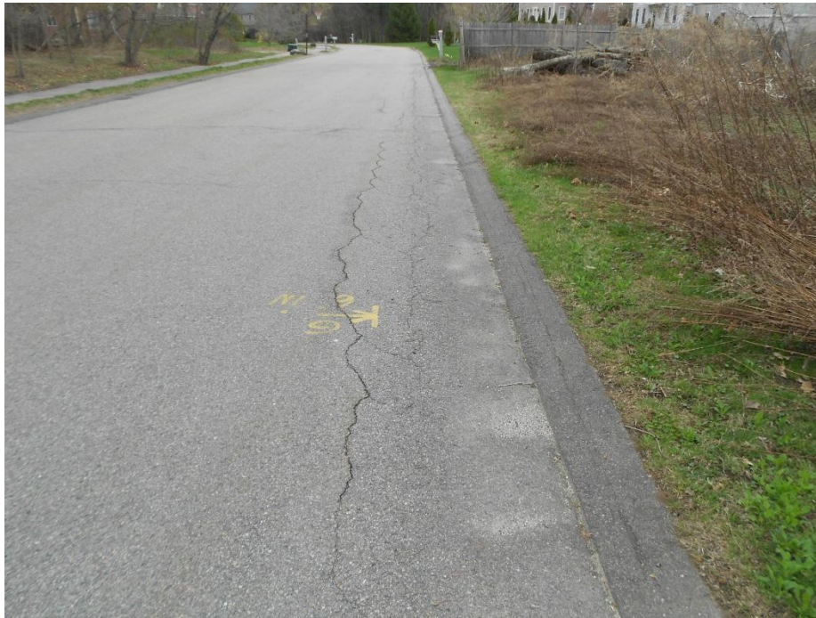
Roadway Cracking
