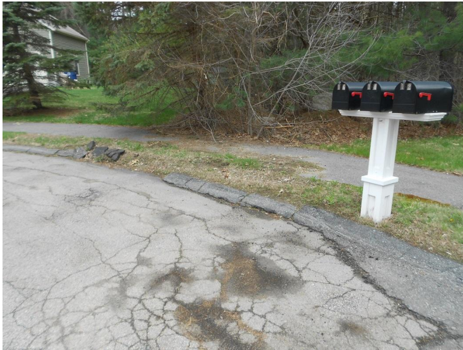
Damaged Berm
