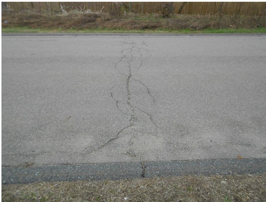
Roadway Cracking
