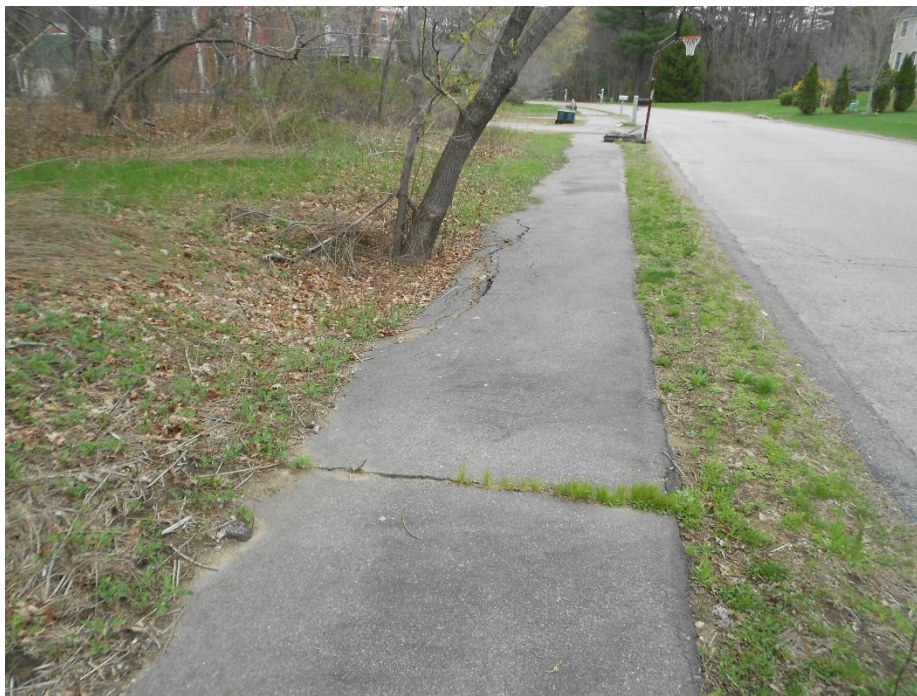
Settling/Cracking Sidewalk
