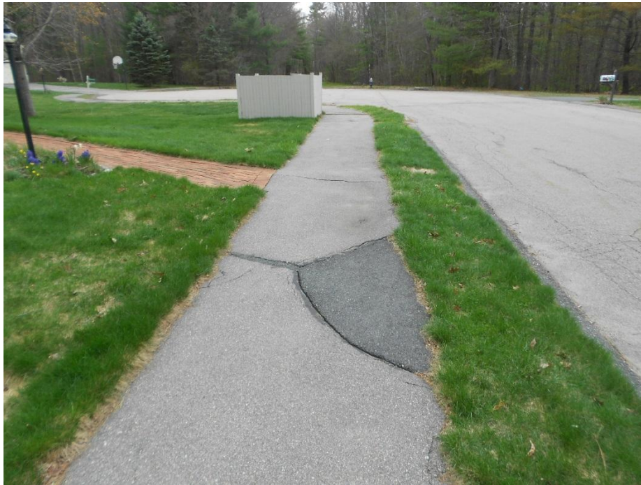
Settling/Cracking Sidewalk
