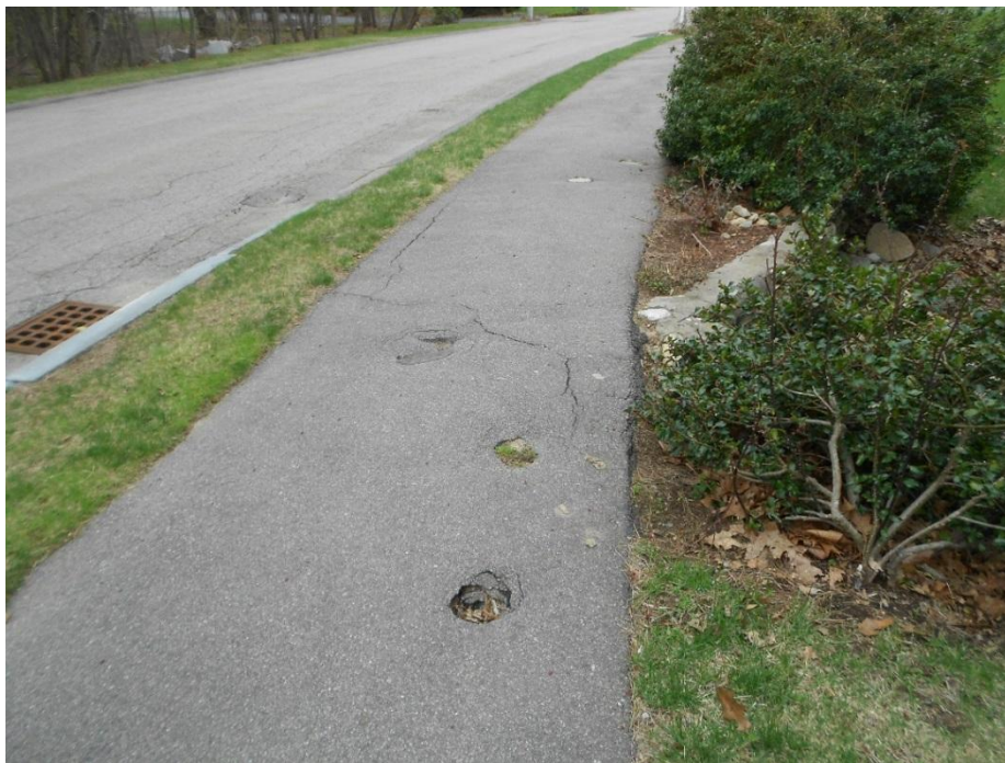
Settling/Cracking Sidewalk
