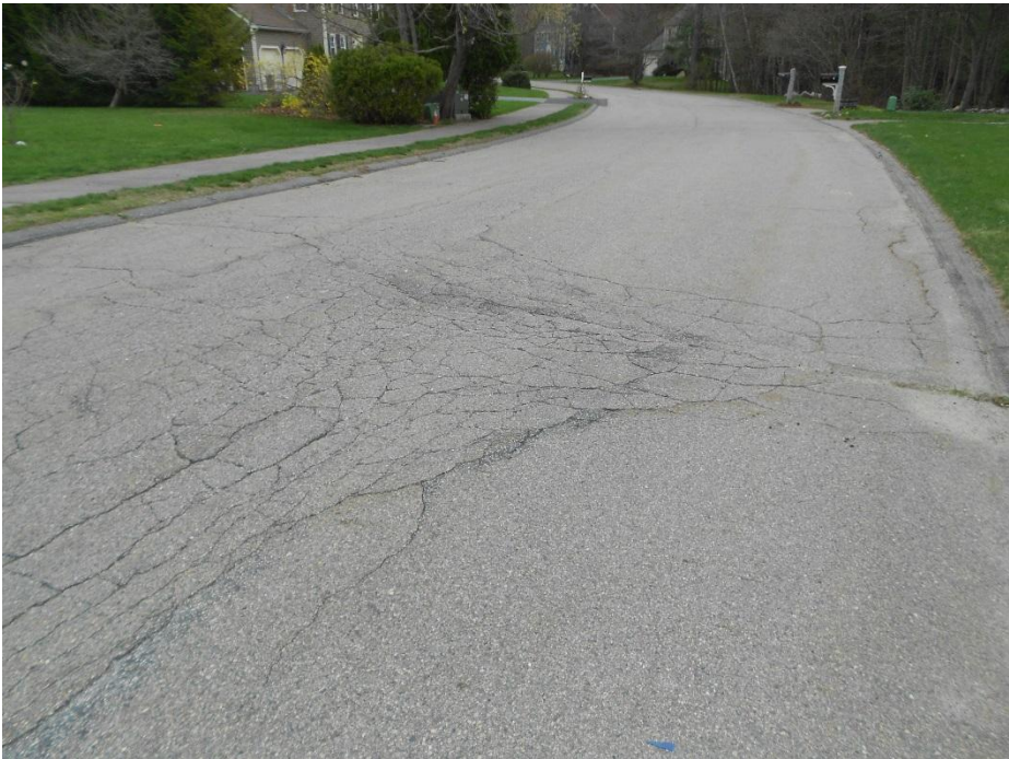
Roadway Cracking
