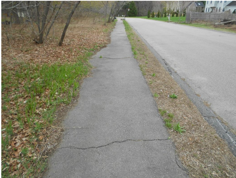
Settling/Cracking Sidewalk
