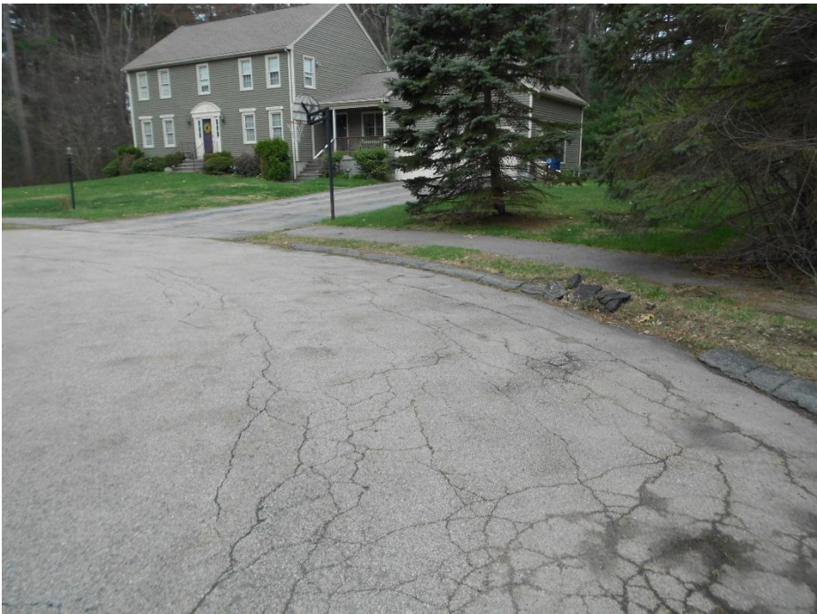
Roadway Cracking
