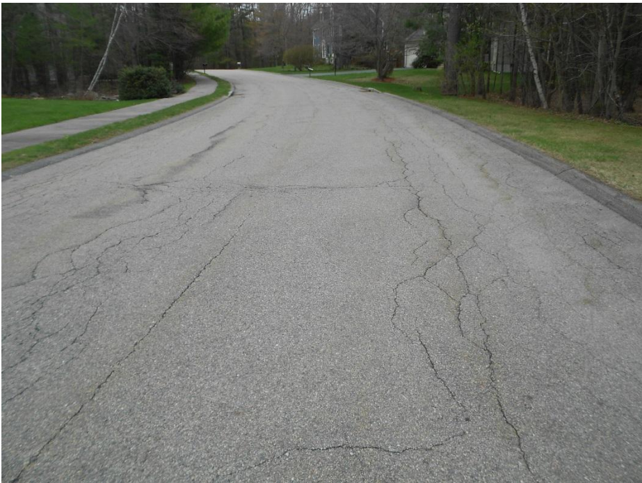
Roadway Cracking
