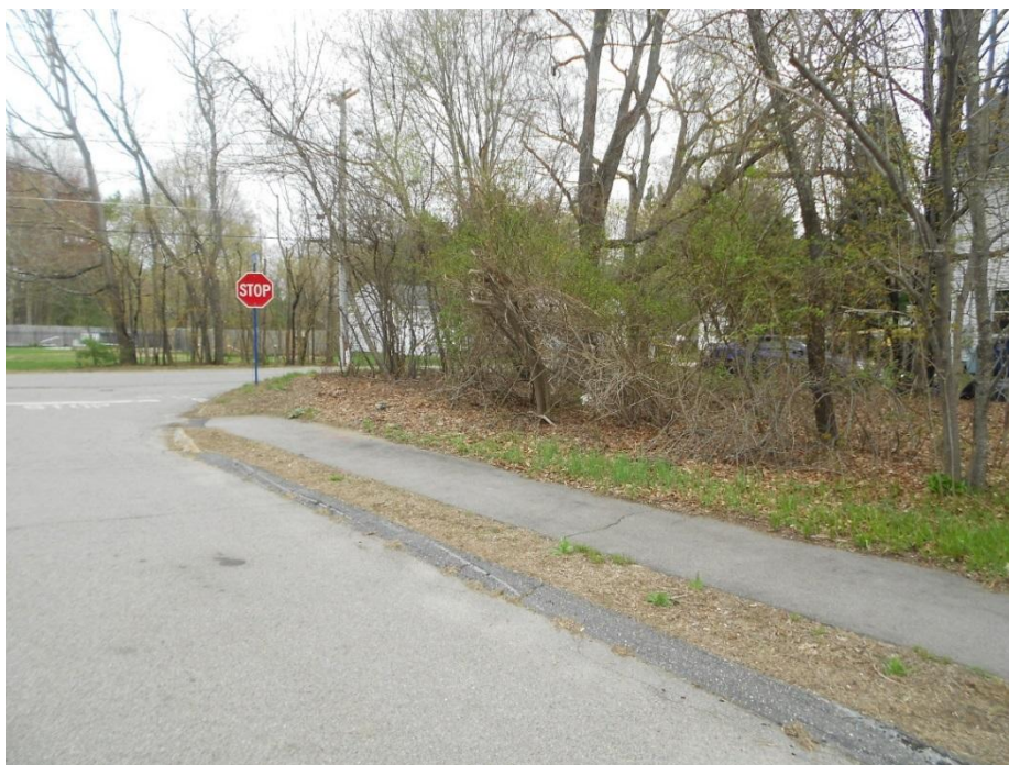
Site Distance Issues from Landscaping/Overgrowth
