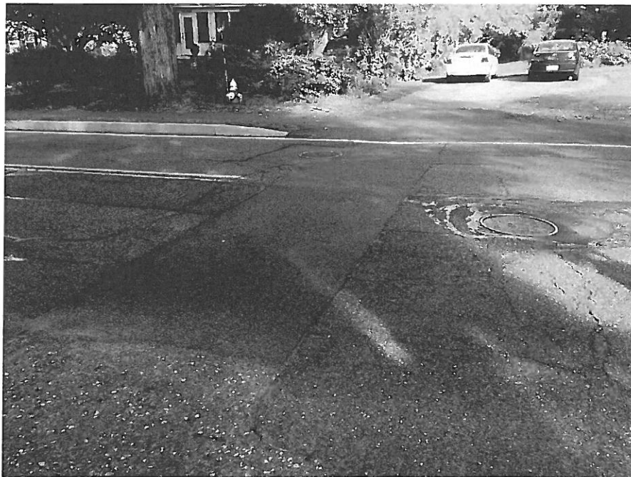
Village Street Water Trench Patch
