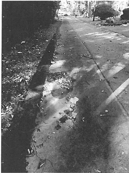
Cherokee Lane Water Trench Patch
