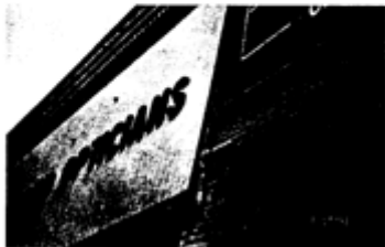
Signs should not cut or overlap wood cornice.
