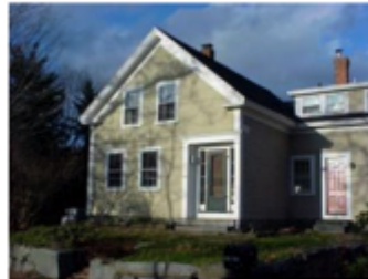
Elevation of buildings should be 2 stories in height above minimized foundation on the front entryway.
