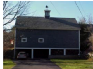
Example of how the elevation below the primary floor line may be differentiated while maintaining the consistency of the basic structure.
