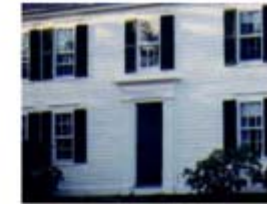
Example of shutters of correct scale and proportion, as well as opening symmetry/rhythm, and window moldings.
