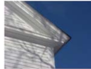
Good example of gable end roof hangover and projection of detail.
