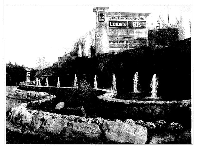
5. Precast and engineered concrete walls, veneered with stone - Note vertical "seam" in stone; wall units may have been engineered and built off-site then crane-placed and co-joined onsite atop foundations. Total height from sidewalk may be 25'H between grade changes across perhaps 40' of horizontal distance. Difficult to imagine something this palatable being proposed but there are options if leveled land mass isn't held to such a premium.
