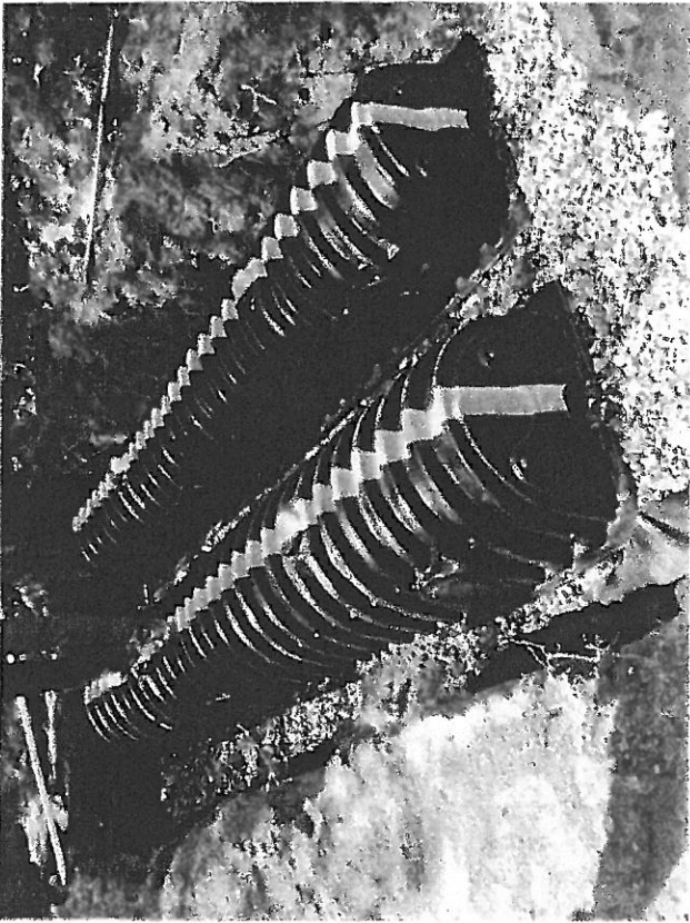
(6-10-13) 10' x 20' Roof Drain Recharge System during install
