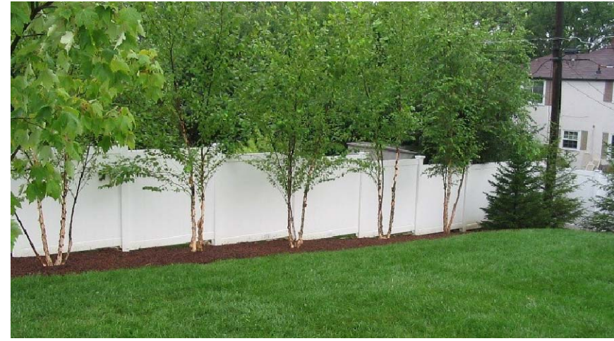
PROPOSED SOLID-PANEL VINYL PRIVACY FENCE HEIGHT VARIES 6' AND 8' (SEE PLAN)
