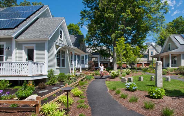
Figure 98: Simple architectural detail reinforces a quality residential development
