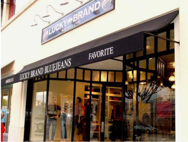
Figure 46: Awning is opaque and integrated into the building façade
