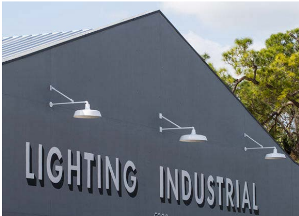
Figure 74: External lighting fixtures that project light onto the sign are strongly encouraged
