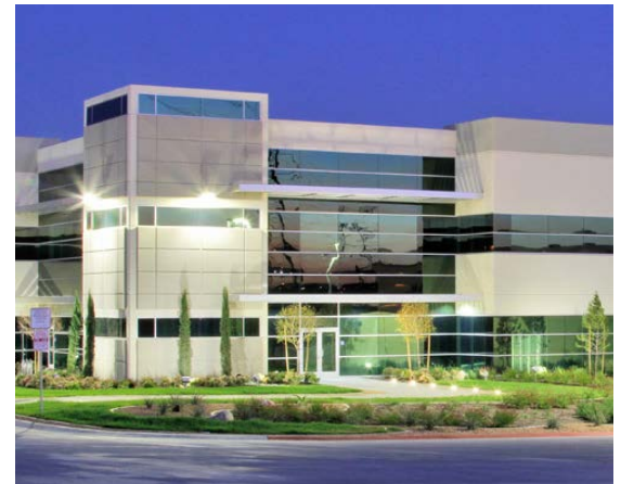
Figure 67: Lighting fixtures contribute to the overall character of the site and building
