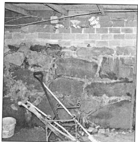
basement was excavated if it did not exist, and new cellar walls of split granite boulders was constructed up to the elevation of the exterior grade. Above grade, the house was underpinned with slabs of granite backed by a veneer of brickwork.
