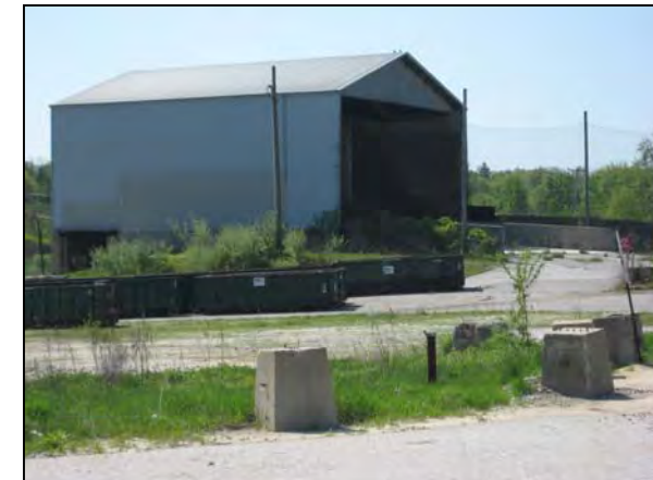
Old Transfer Station located along Rt. 28 Source: SNHPC
