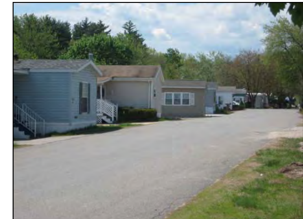
View of Bockmon Mobile Home Park
