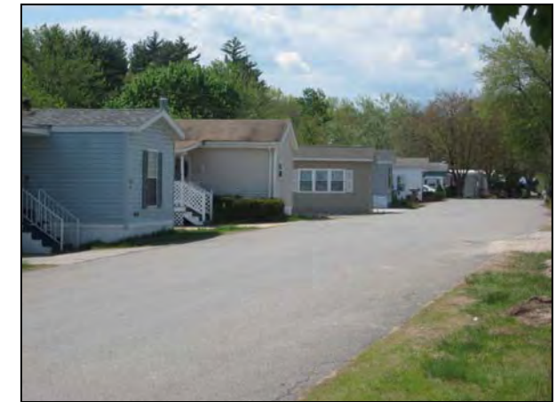
View of Bockmon Mobile Home Park
