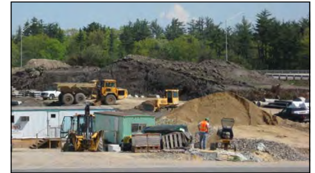
Construction at Exit 5 on I-93 Source: NH DOT
