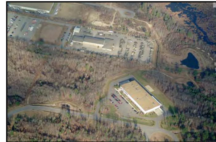
US. Army Reserves and FCI Electrical Power Interconnect Division Source: SNHPC
