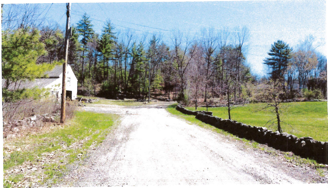
Description: Additional barn near the end of Page Rd which is a class VI road.
