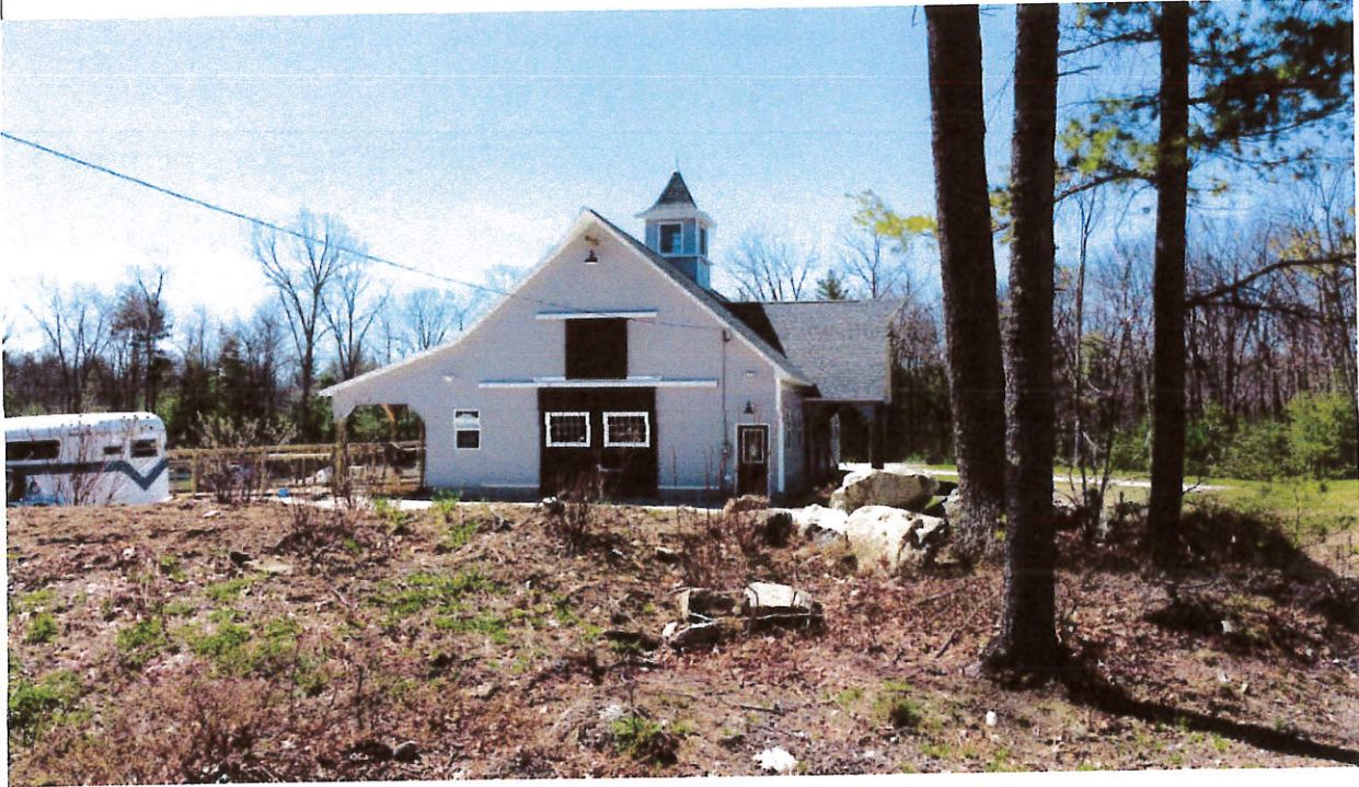
Description: Side view of the barn on Page Rd which is also a class VI road.
