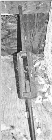
*Left: Typical turnbuckle installed to link wall plates (top) with beams below (one of four).*
