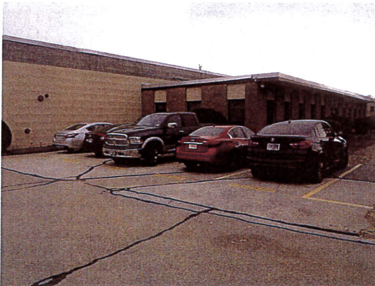
Existing northern and western façade and area of proposed 900-sf office addition (paved area to be removed), looking southeast from paved parking area
