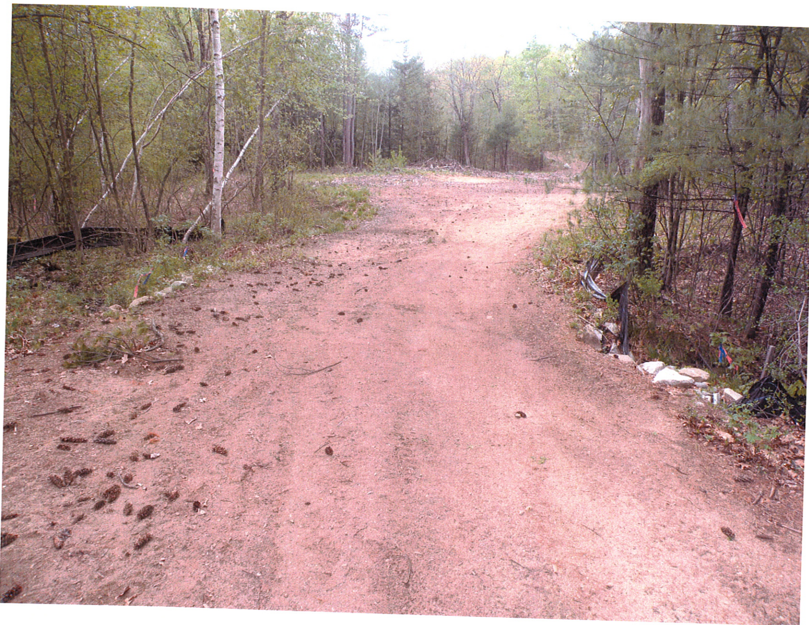
Culvert crossing Wetland B1
