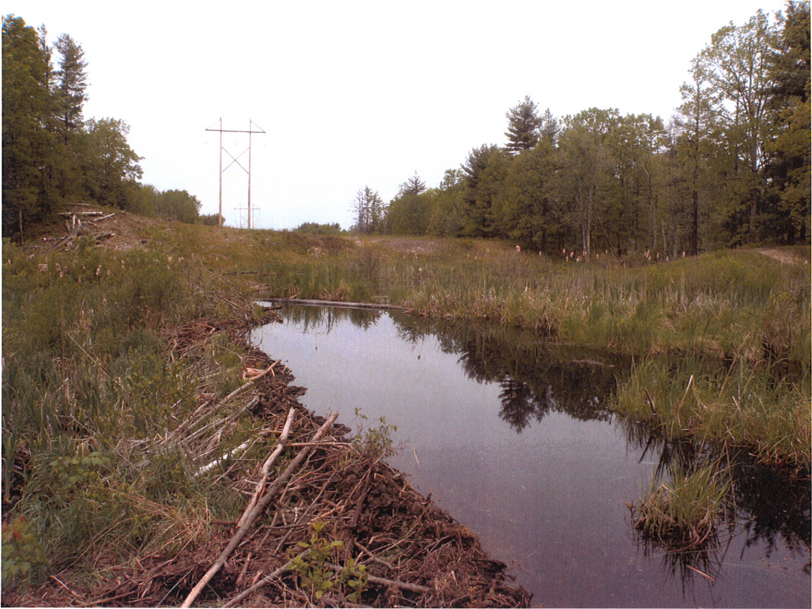
Dam at Wetland X2 left and X4 right
