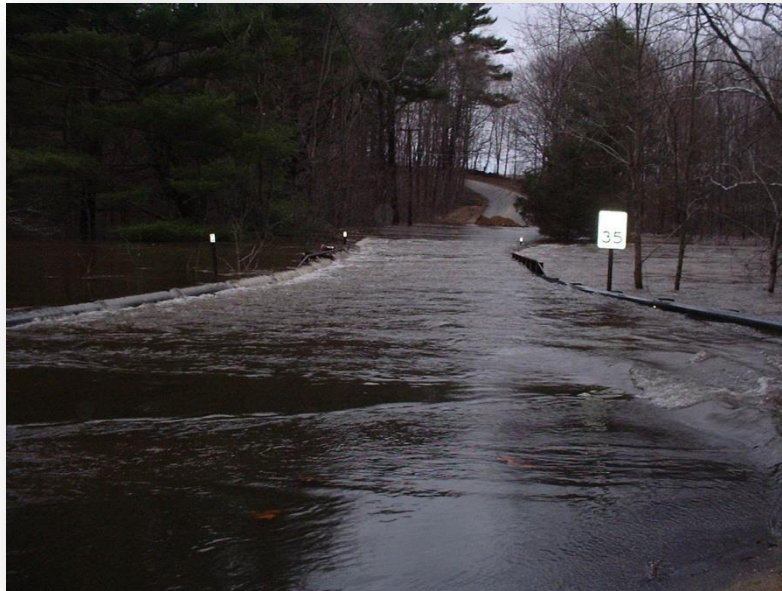
High Road Bridge, May 2006 Flooding Event
