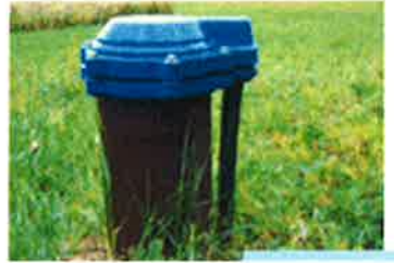
Drilled Bedrock or Point Driven Well
