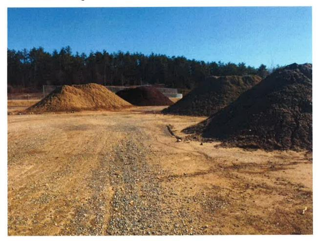
Step 2- Spread and grade out the piles shown below in this picture to fill in the sags, hollows, and low spots to level the area off. The material is kind of a loamy fill.
