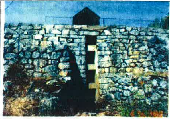
Downstream face and outlet works of Mendums Pond Dam
