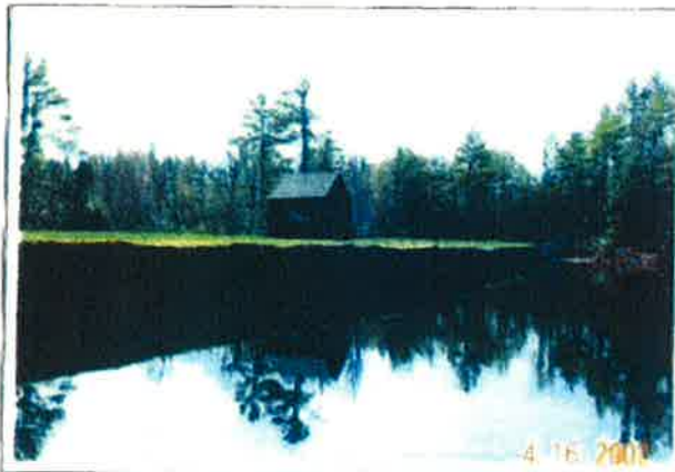
Upstream Face of Mendums Pond Dam at full lake level
