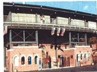
Nashua, NH Holman Stadium Reconstruction
