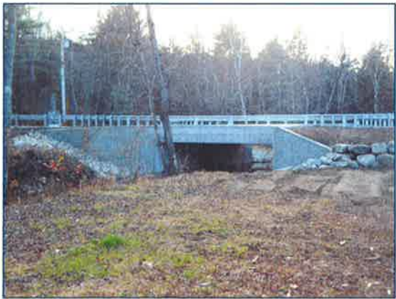
Warmac Road Bridge – Swanzey, New Hampshire
