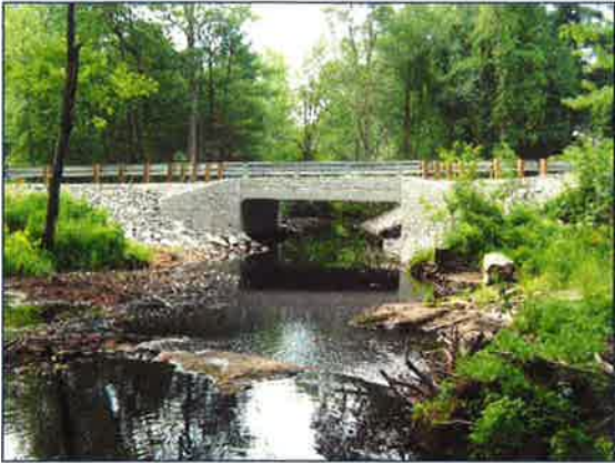
Drew Road Bridge over Drew Brook – Derry, New Hampshire
