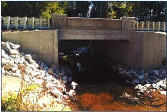
Shannon Road Bridge – Salem, New Hampshire
