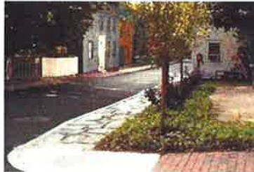
Portsmouth, NH Lower Court Street Reconstruction
