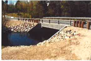
New Durham, NH Davis Crossing Road over Ela River
