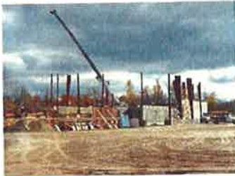
Merrimack, NH Transfer Station
