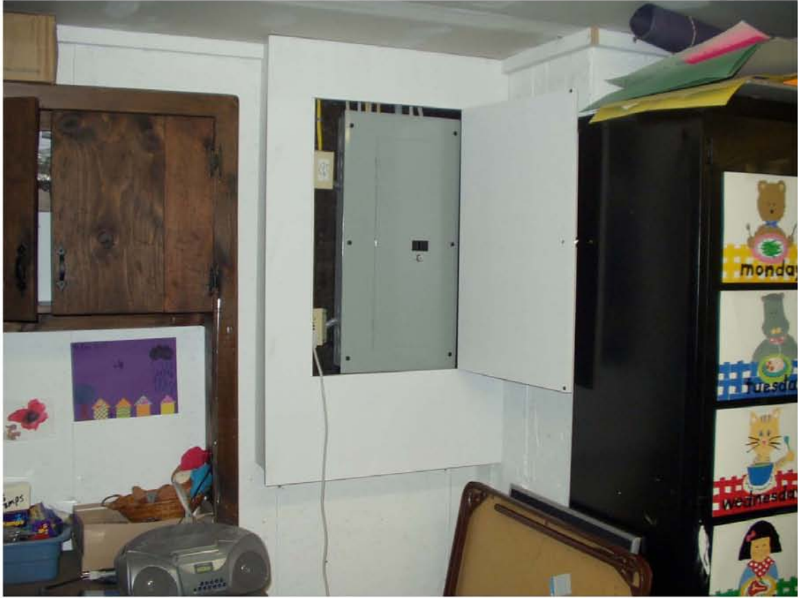
HISTORICAL SOCIETY UPSTAIRS LIGHTING
