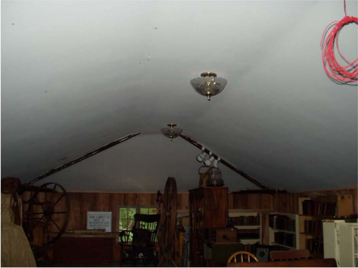
ANNEX FIRE ALARM MAIN PANEL AND ELECTRICAL SERVICE PANEL (AND QUESTIONABLE WIRING)
