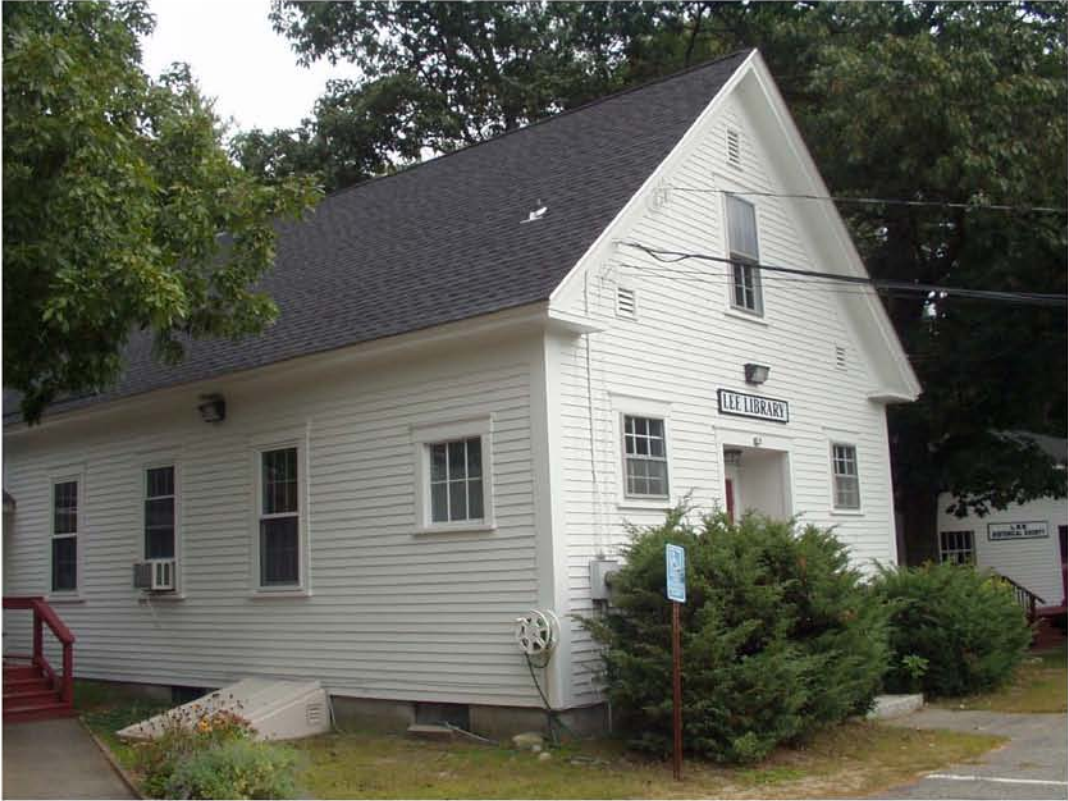
LIBRARY SERVICE ENTRANCE AND METER
