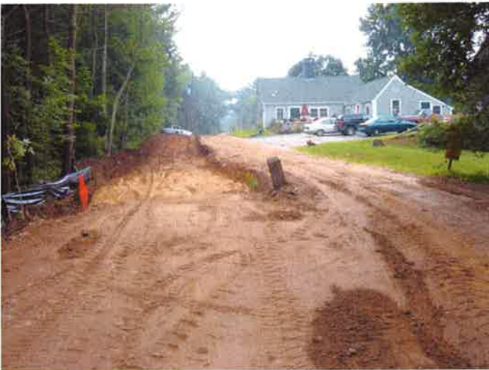
DURING ROAD WIDENING
