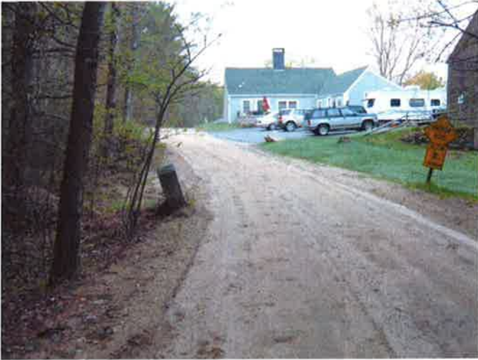
BEFORE ROAD WIDENING
