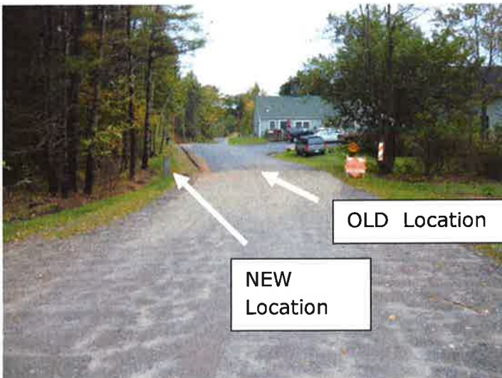
AFTER ROAD WIDENING
