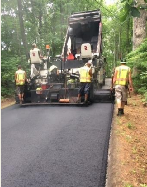
PAVING YORK LANE
