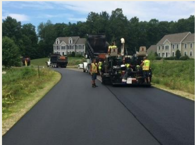
PAVING THURSTON WOODS
