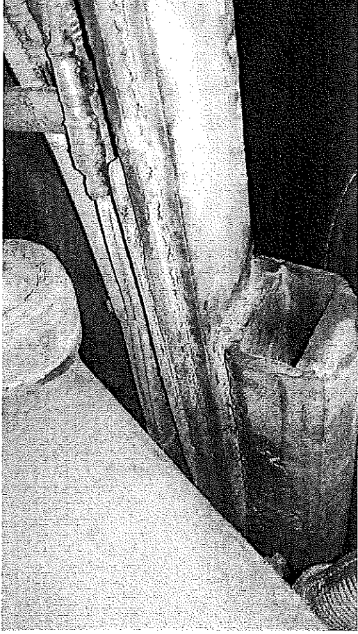
Pictures of Frame Corrosion Being Repaired Under Warranty
