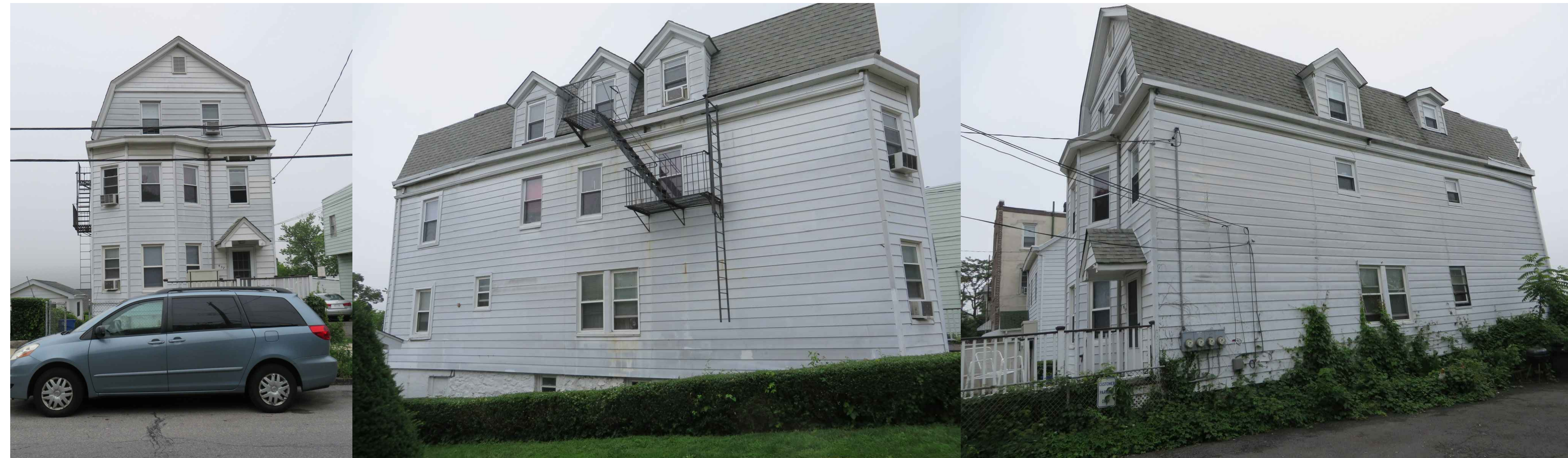
VIEWS OF EXISTING HOUSE at 457 WARBURTON AVENUE SCALE: N.T.S.
