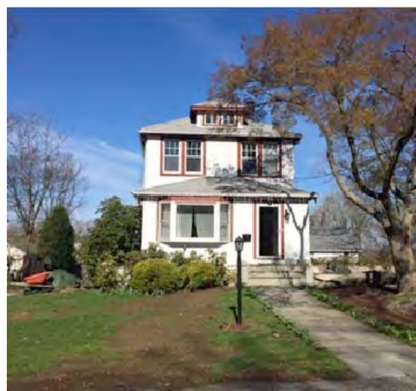
83 COCHRANE AVE (front view)
