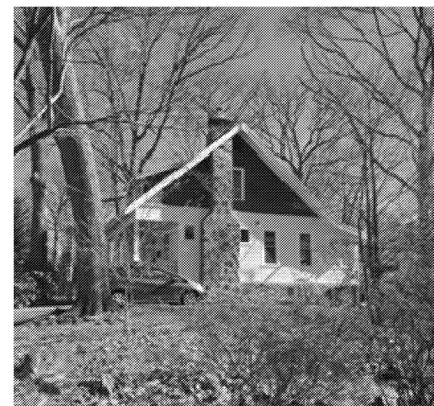
74 COCHRANE AVE (front view)
