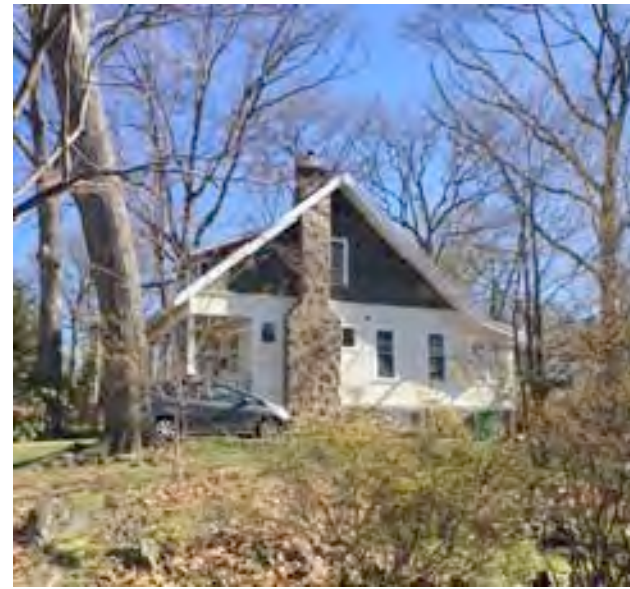
74 COCHRANE AVE (front view)
