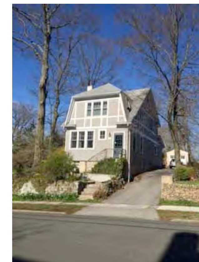
19 LEFURGY AVE (side view)
