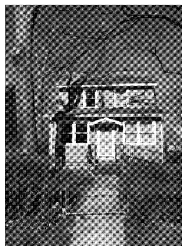
77 COCHRANE AVE (front view)
