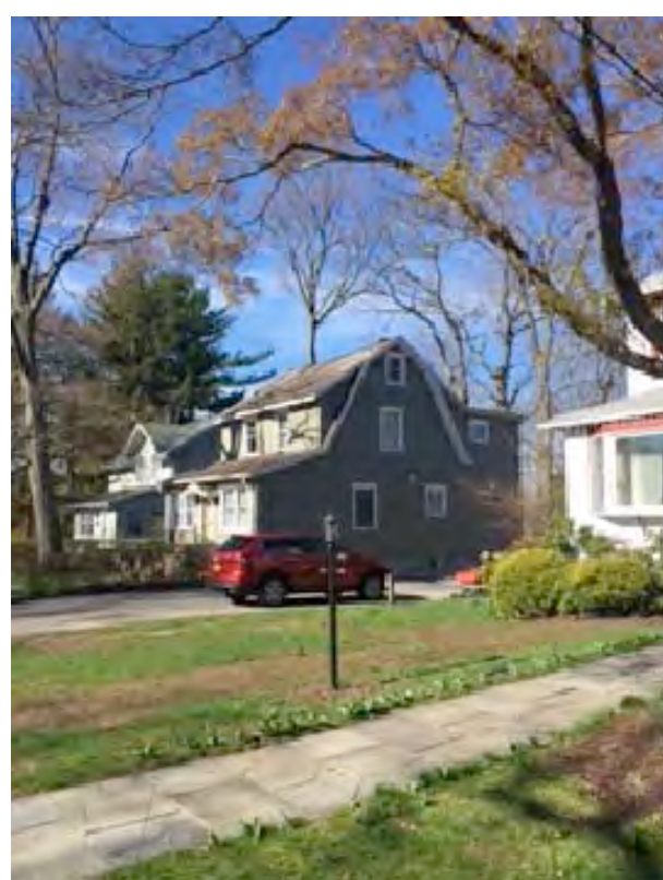
77 COCHRANE AVE (side view)
