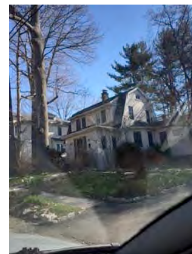
62 COCHRANE AVE (side view)
