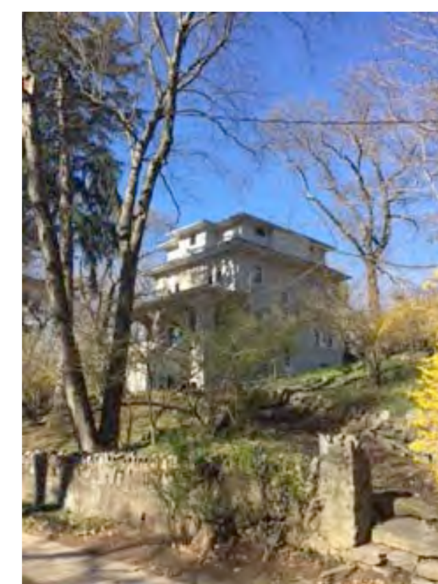
39 LEFURGY AVE (side view)
