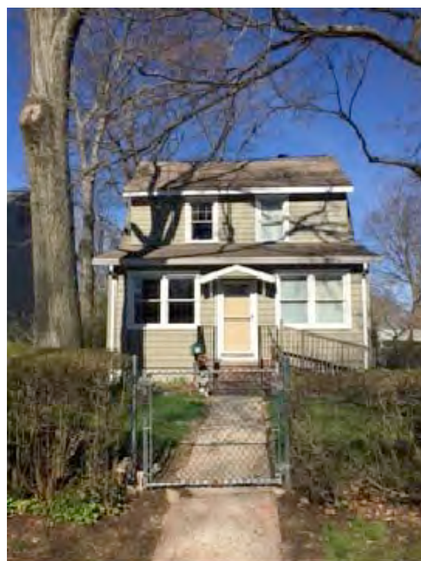
77 COCHRANE AVE (front view)
