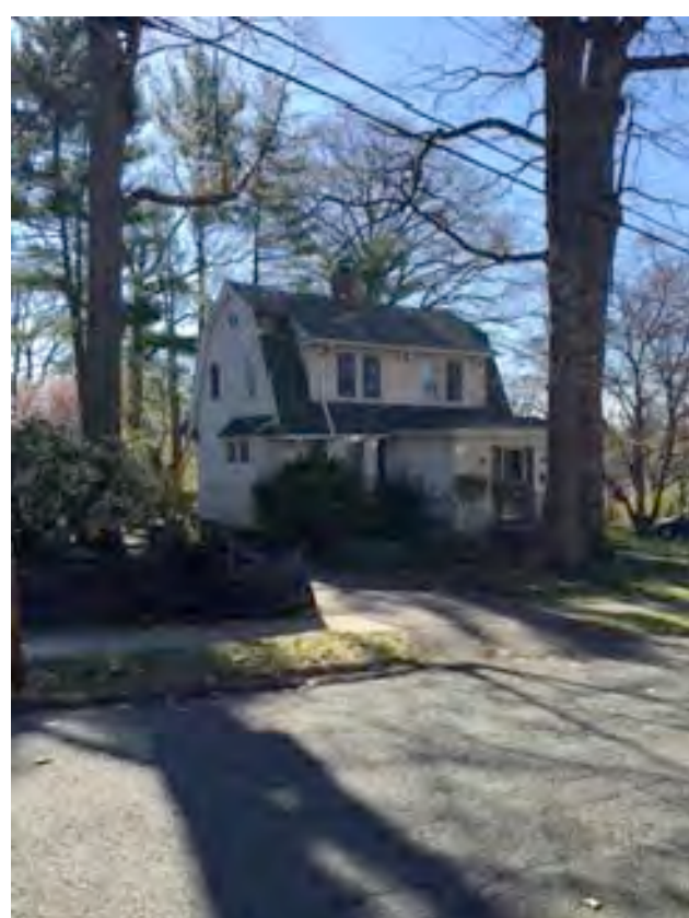
62 COCHRANE AVE (front view)
