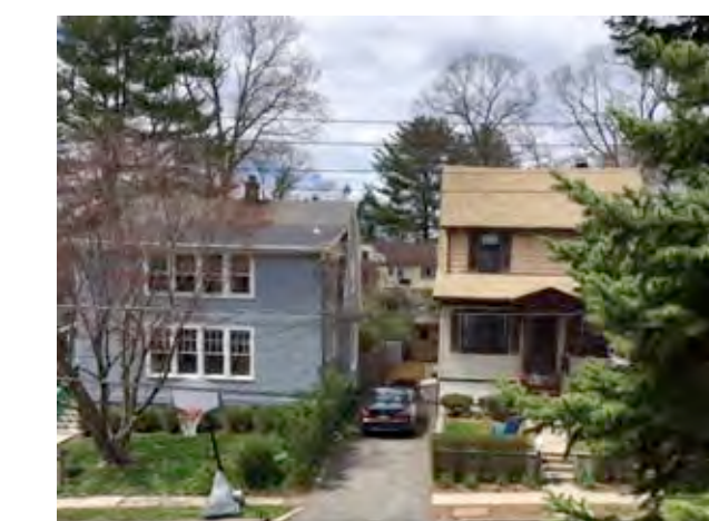
7 LEFURGY AVE (side view)
