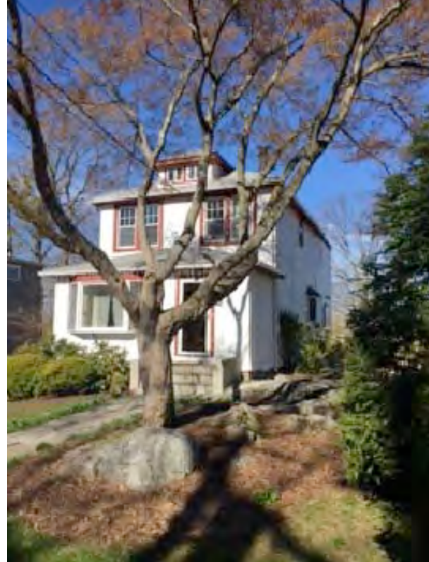
83 COCHRANE AVE (side view)
