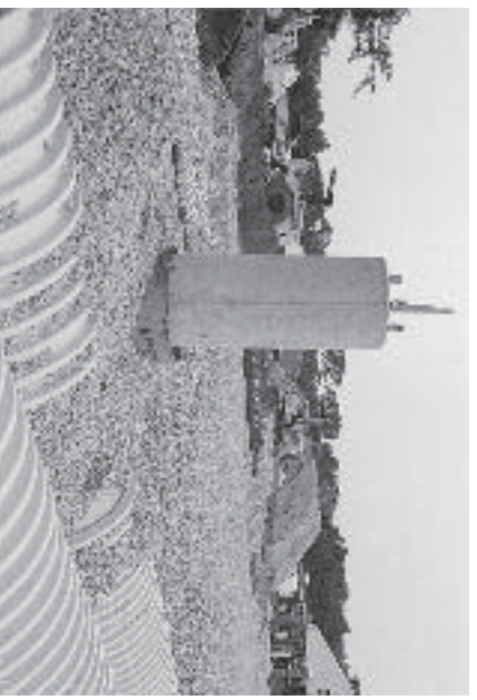
Figure 15 – Chamber bed placed around light post.
