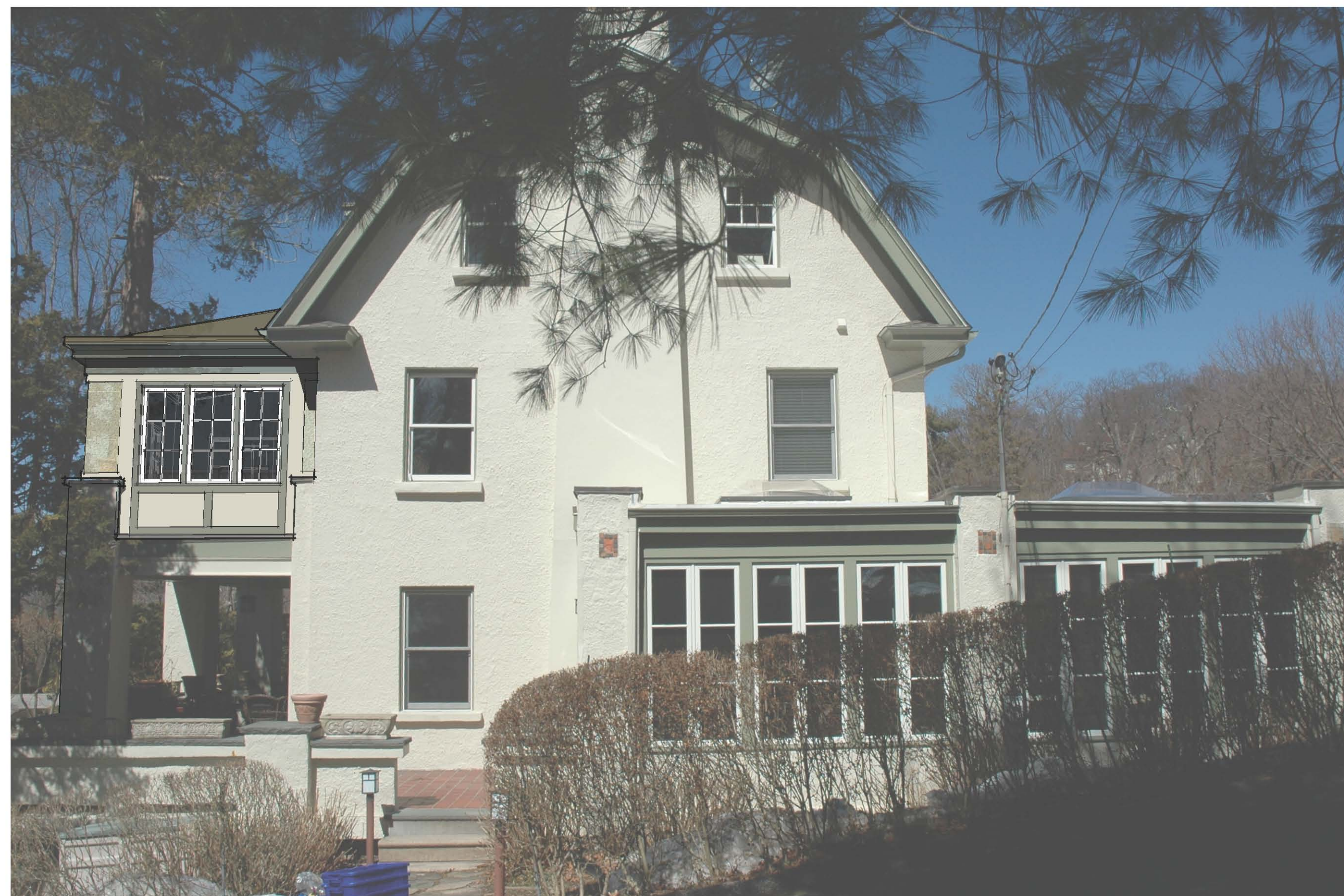
3 SOUTH ELEVATION VIEW
