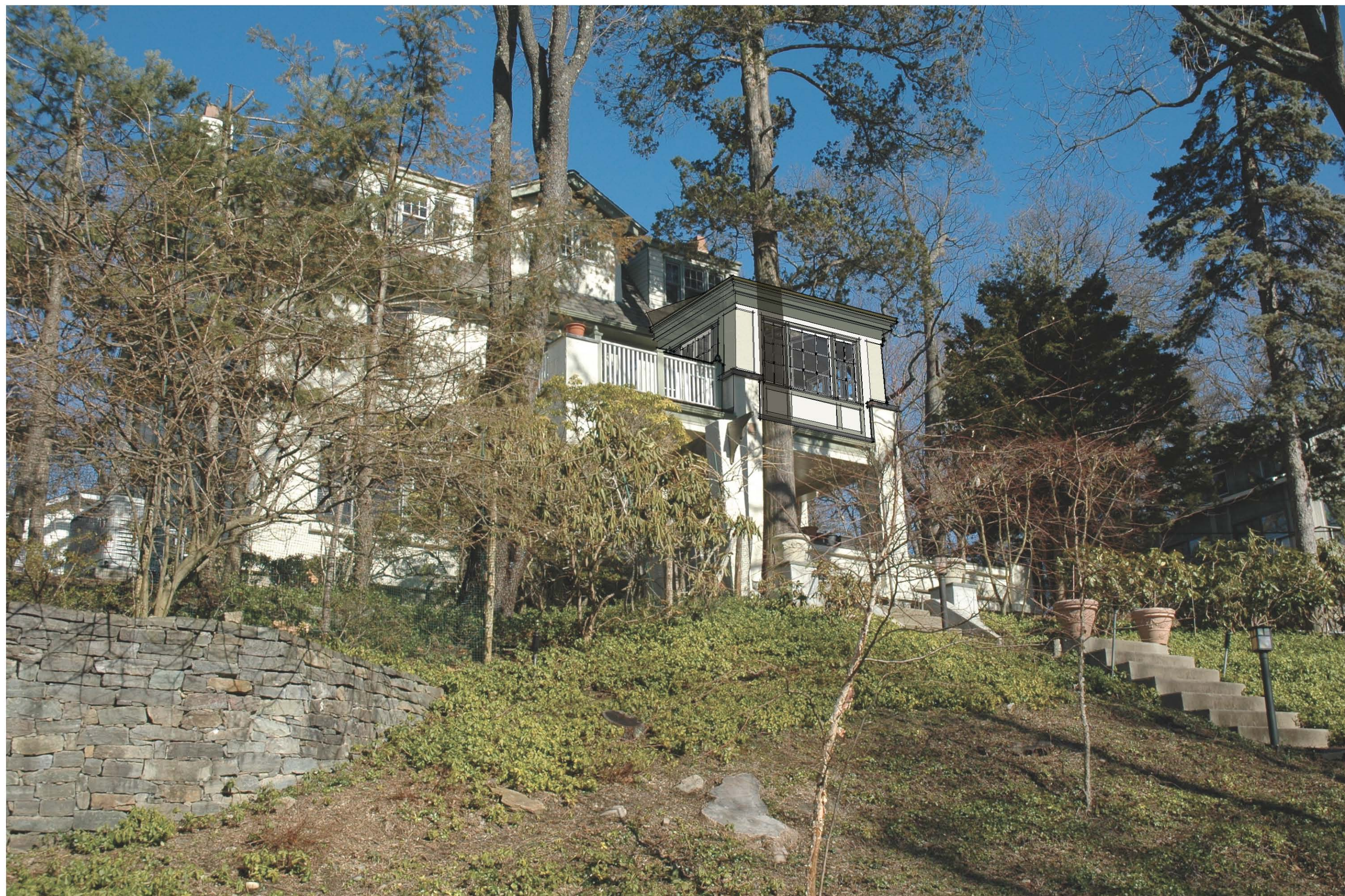
1 NORTHWEST VIEW FROM CIRCLE DRIVE 25 CIRCLE DRIVE HASTINGS-ON-HUDSON, NY 10706
